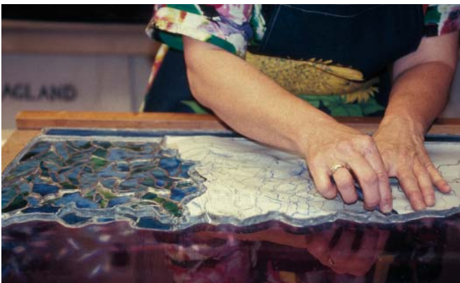
Figure 14. The external glass plate has been removed to clean the interlayer of this plated Tiffany Studios window.
