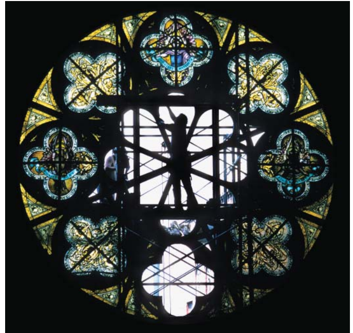
Wooden frame of the rose window undergoing repair (exterior view).
