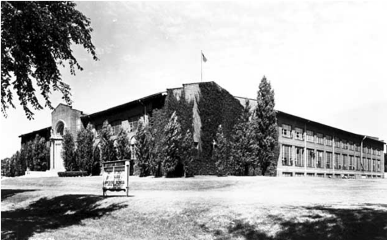
Figure 6.10 The Dunwoody Industrial Institute, constructed in 1917, provided private vocational and technical training for Minneapolis residents during the Modern Era. Dunwoody Industrial Institute, November 10, 1942. Norton & Peel Photograph Collection, Minnesota Historical Society.
