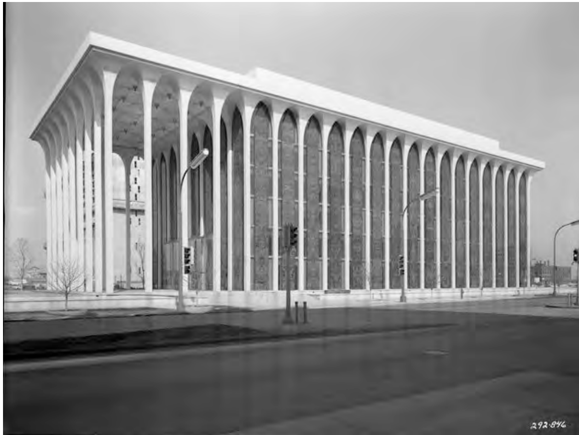
Figure 4.5 The Northwestern National Life Building, designed by Minoru Yamasaki, was constructed in 1964. Northwestern National Life Building, 1965. Norton & Peel Photograph Collection, Minnesota Historical Society Collections Online.
