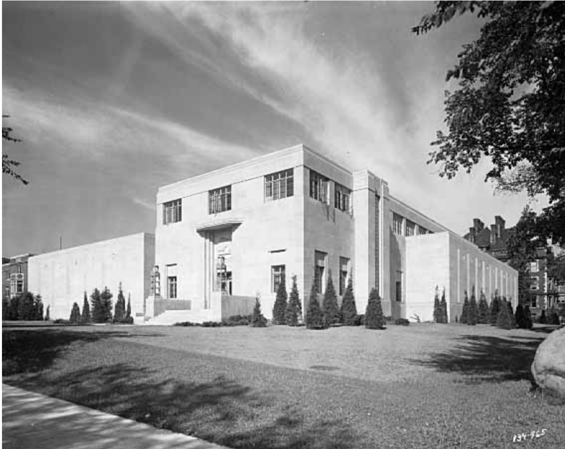
Figure 2.2 The PWA was responsible for the construction of the Bell Museum of Natural History at the University of Minnesota. The recessed windows, smooth stone sheathing, low relief sculptural elements all help identify this building as designed in the PWA Moderne style. University of Minnesota Bell Museum of Natural History, July 27, 1940. Norton & Peel Photograph Collection, Minnesota Historical Society.
