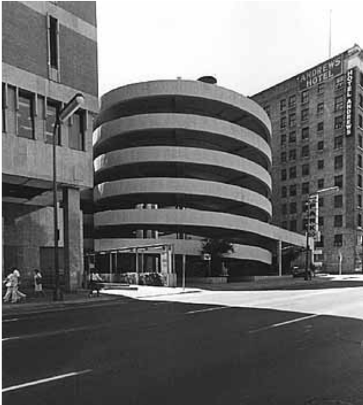
Figure 3.9 This corkscrew-style ramp was one of the more distinctive private ramps constructed downtown after World War II.
