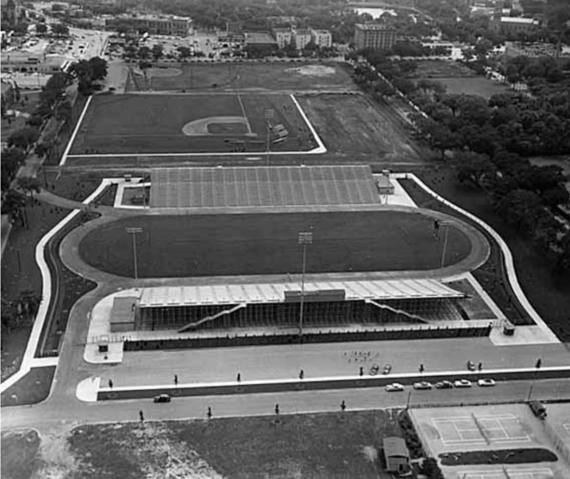
Figure 8.10 Parade Stadium, constructed at Parade park in 1951, provided a venue for high school football games during the 1950s and 1960s. Other athletic facilities at the Parade are visible in the foreground and background. Parade Stadium, July 17, 1952. Minnesota Historical Society.
