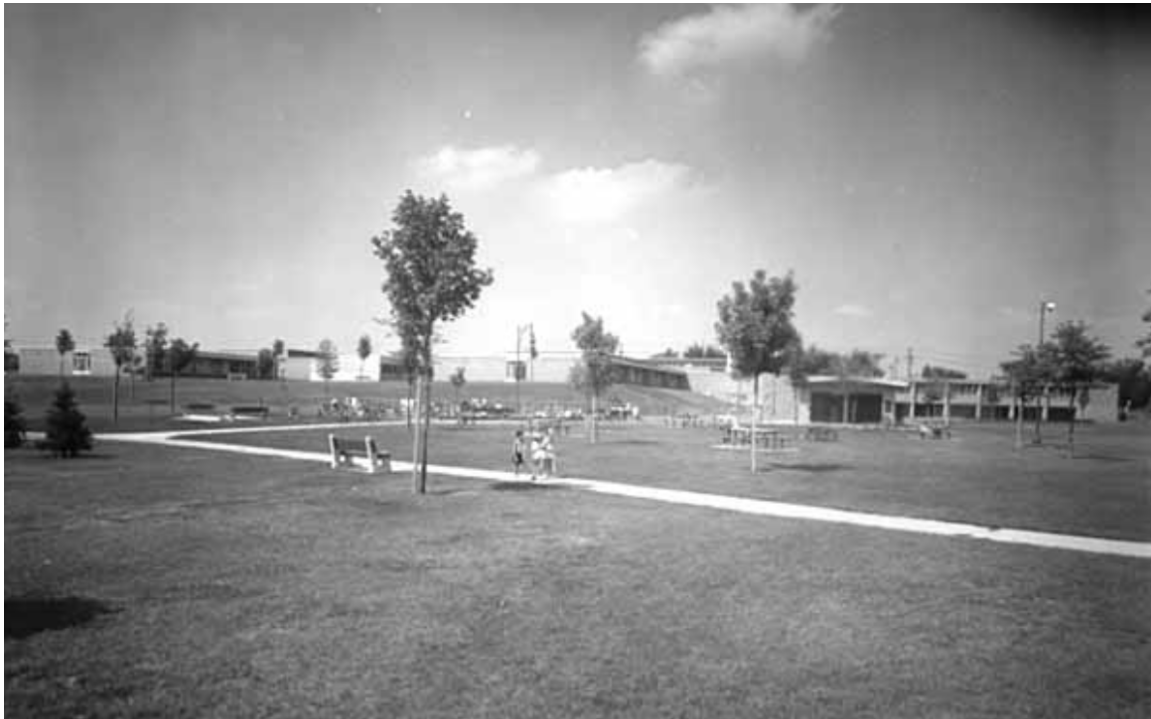
Figure 6.4 Armatage Elementary School, constructed in 1952, featured a 23-acre landscaped site. Armatage Elementary School, August 11, 1958. Norton & Peel Photograph Collection, Minnesota Historical Society.
