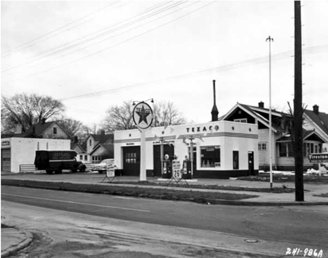
Figure 8.1 The design of this Texaco service station at 3744 Fifteenth Avenue South reflects the white oblong-box style that became popular for chain service stations beginning in the late 1930s. 3744 Fifteenth Avenue South, November 30, 1956. Norton and Peel Photograph Collection, Minnesota Historical Society.
