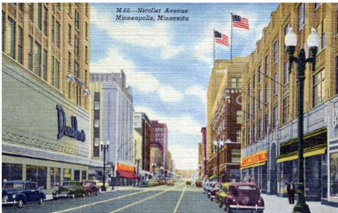
Figure 3.5 During the 1940s and 50s, some downtown businesses modernized their façades by replacing storefronts or adding a second layer of cladding material. The renovated façade of Donaldson's Department Store on Nicollet Avenue is visible at the left of the postcard. Postcard of Nicollet Avenue, 1958. Lakeswoods Postcard and Postcard Image Collection, Lakeswoods.com.
