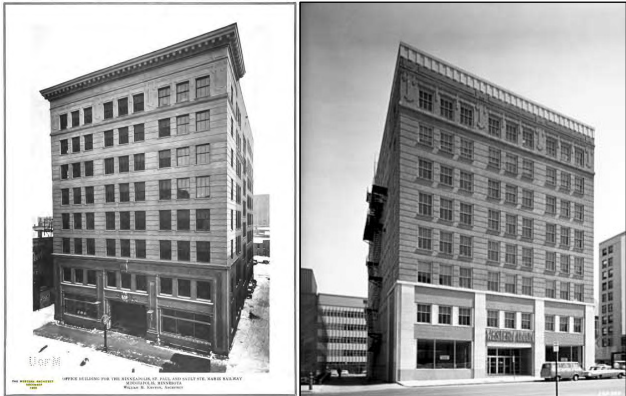
Figure 4.6 The original Soo Line Office Building (later known as the Western Union Building), 317 Second Avenue South (William M. Kenyon, original building 1909; façade modernization, architect unknown, 1962) before and after 1962 façade modernization that simplified the building’s cornice, and storefront systems.
