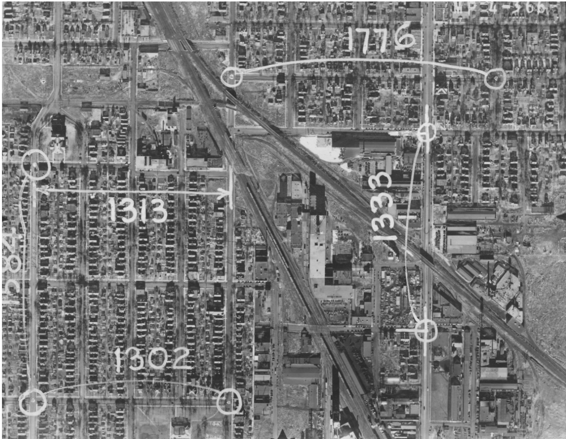
Figure 3.1 During the 1930s, some industrial firms were located along railroad lines in outlying areas of Minneapolis, such as the intersection of the Great Northern and the Northern Pacific Railways in Northeast Minneapolis. Aerial view of industrial plants along the Great Northern Railway and the Northern Pacific Railway, 1938. John R. Borchert Map Library, University of Minnesota.
