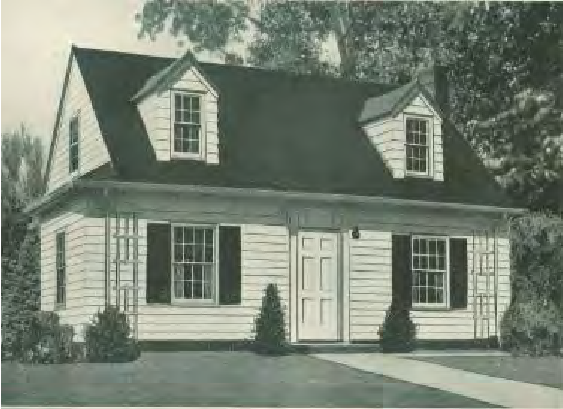
Figure 5.3 During the immediate postwar era, small, compact houses such as the Cape Cod shown above were constructed in suburban subdivisions.
