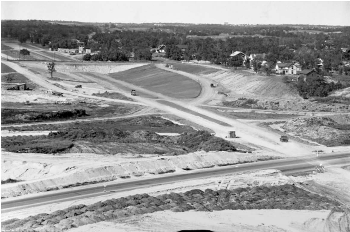
Figure 4.9 The construction of the “Beltline” (Highway 100) around the Twin Cities was financed in part by the Works Progress Administration. Construction of the Beltline Highway (Highway 100), St. Louis Park, Minnesota, August 17, 1937. Minneapolis Star Journal , Minnesota Historical Society.
