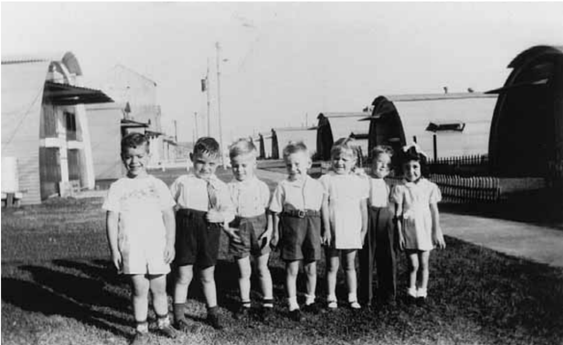
Figure 5.1 After World War II, temporary housing such as this group of Quonset huts was constructed in the Twin Cities to house returning veterans and their families. Quonset huts at Buchanan Street Northeast, c. 1946. Minnesota Historical Society.
