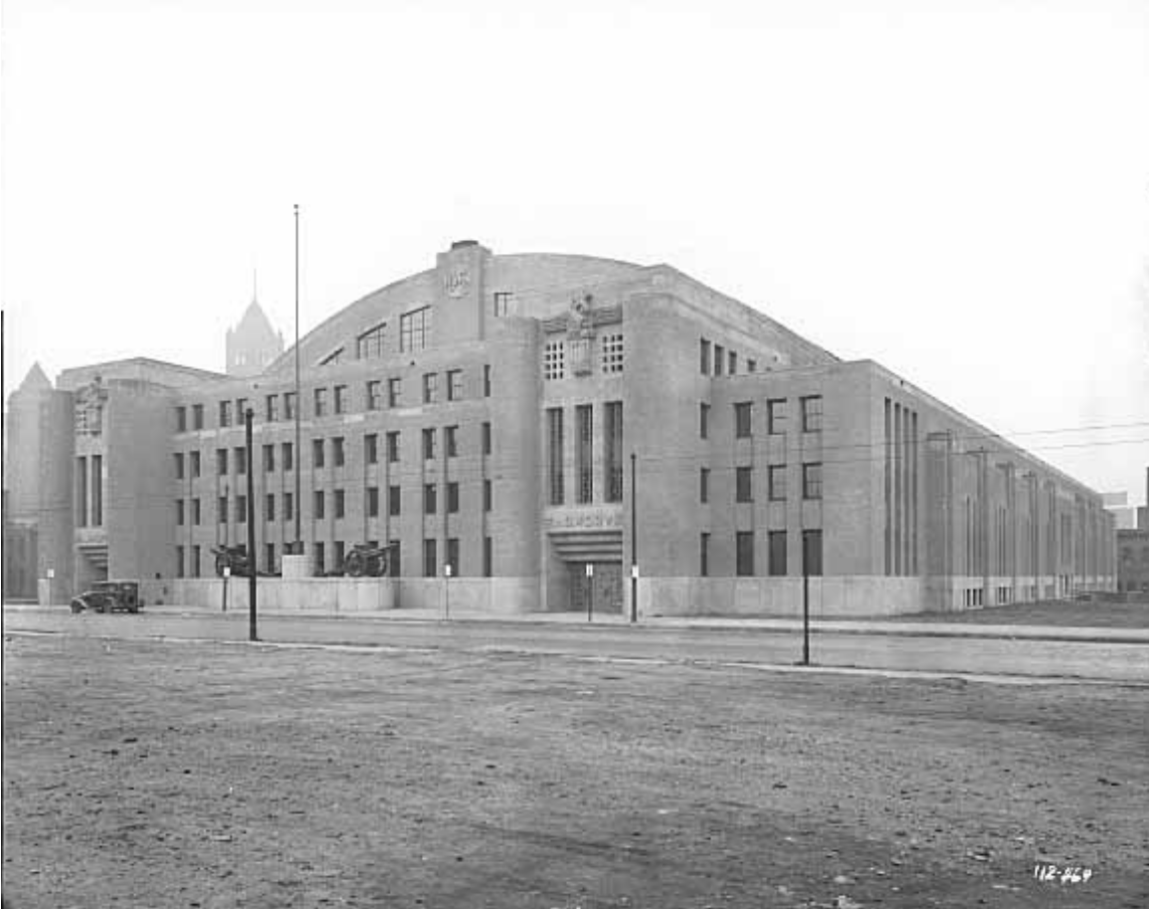
Figure 2.4 The Minneapolis Armory with its symmetrical form, arrangement of piers and recessed vertically stacked windows, smooth stone sheathing, and interior murals is an excellent example of the PWA Moderne style. Minneapolis Armory, November 13, 1935. Norton & Peel Photograph Collection, Minnesota Historical Society.
