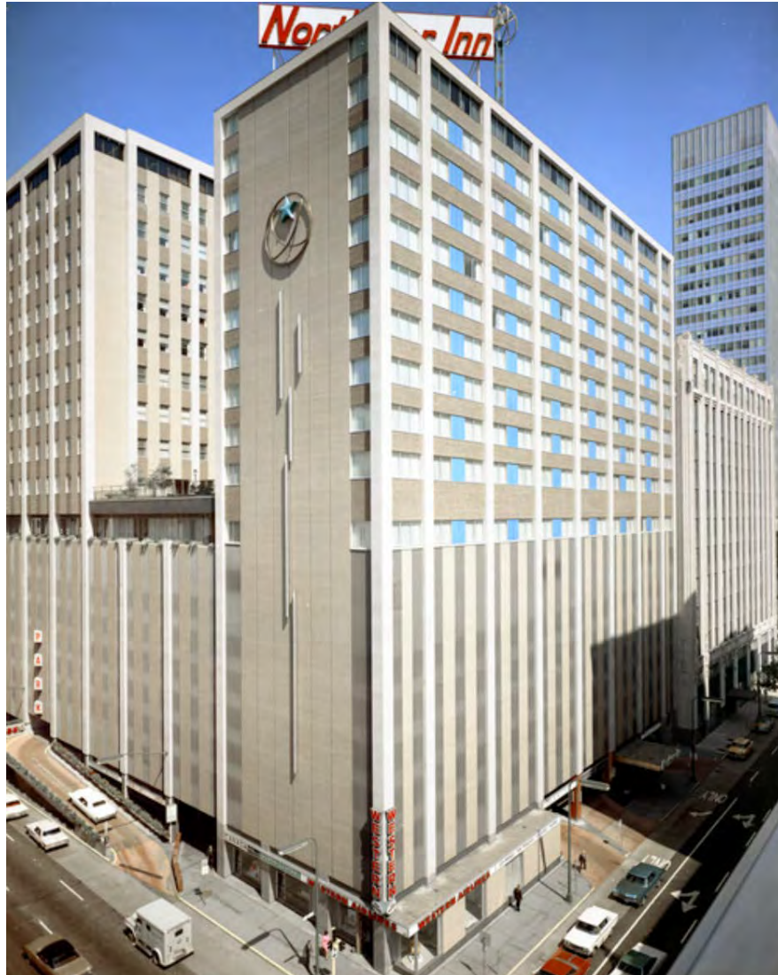
Figure 3.10 Northstar Center, constructed in 1962, featured the first skyway in Minneapolis, as well as an elevated courtyard and two nine-story towers set above a parking ramp. Northstar Center, 1967. Norton & Peel Photograph Collection, Minnesota Historical Society.
