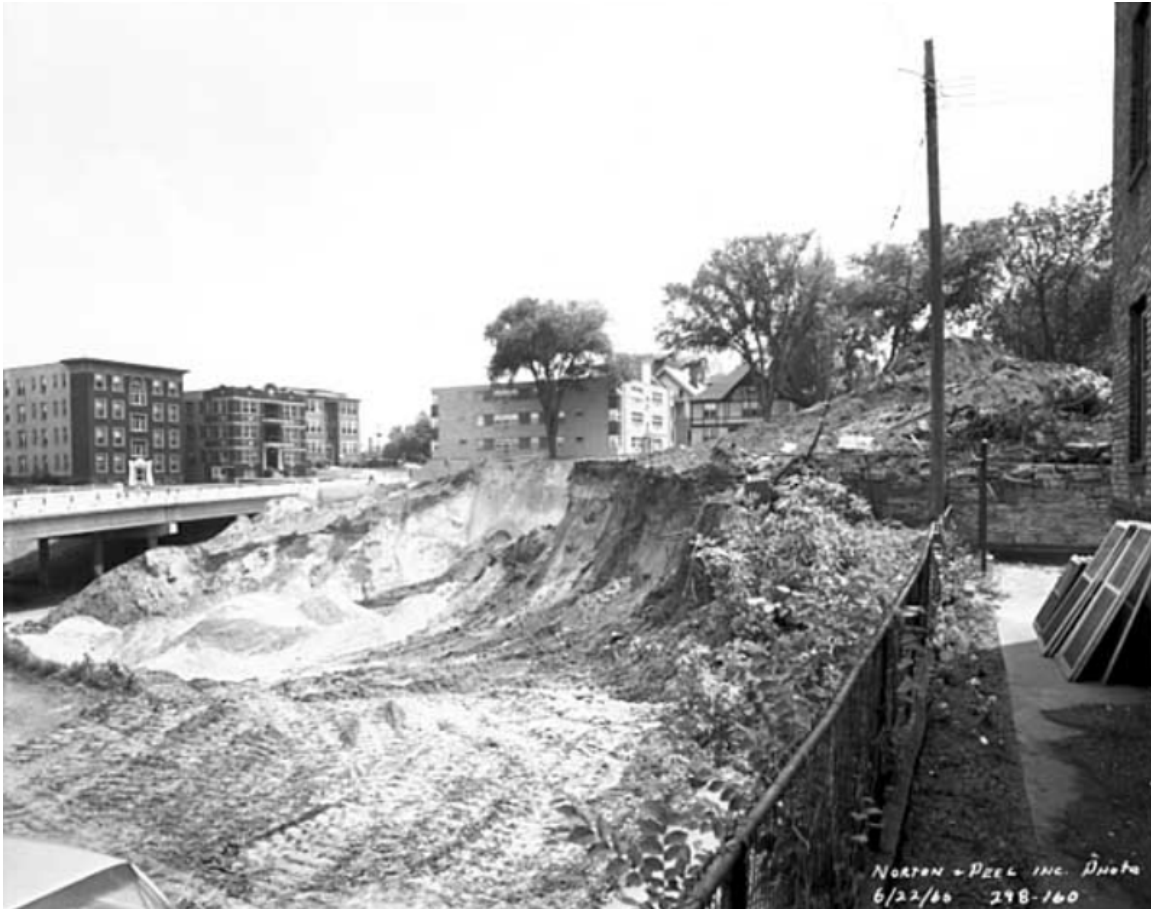
Figure 4.12 The 11-mile segment of Interstate 94 from Hennepin and Lyndale Avenues in Minneapolis to Marion Street in St. Paul (including the section shown here) opened in 1968. Construction of Interstate 94 looking towards Blaisdell Avenue in Minneapolis, June 22, 1966. Norton & Peel Photograph Collection, Minnesota Historical Society.
