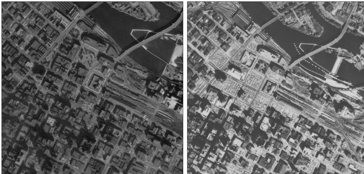
Figure 4.1 The Gateway District before and after demolition. Aerial photographs from 1957 (left) and 1964 (right).
