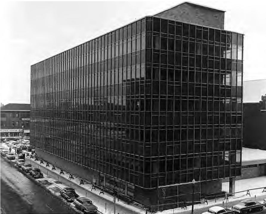
Figure 9.5 Lutheran Brotherhood Building, nearing the end of construction in 1955.
