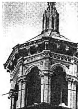
Figure 9. Exterior of the Lantern from the Pistoia Baptistery, (finished 1359).
