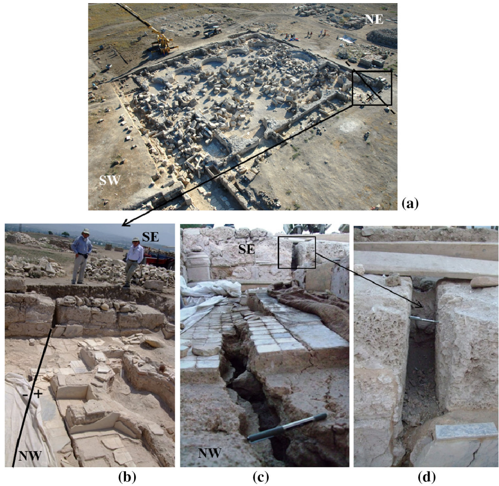
Fig. 11 Damages of Laodikeia Church after the seventh century AD earthquake: a unearthed collapsed structure (Laodikeia 2013), b–d surface ruptures at the east corner of the Laodikeia Church structure
