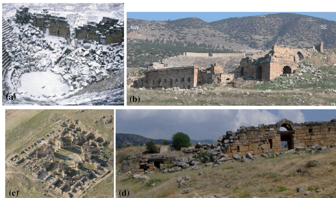
Fig. 8 a, b Damages at the great theatre of Hierapolis after historical earthquakes (location 7) (from Pamukkale 2009), c collapsed view of St. Philip's Martyrium built in early fifth century AD, d damaged part of the city wall at location 9
