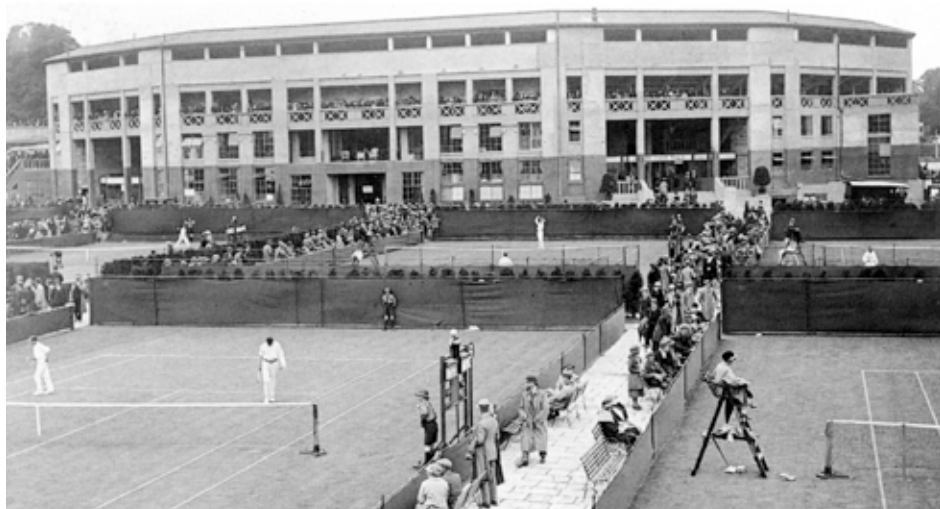
Above: The newly built Centre Court is pictured during The Championships 1921, several years before the Boston Ivy enveloped its exterior
