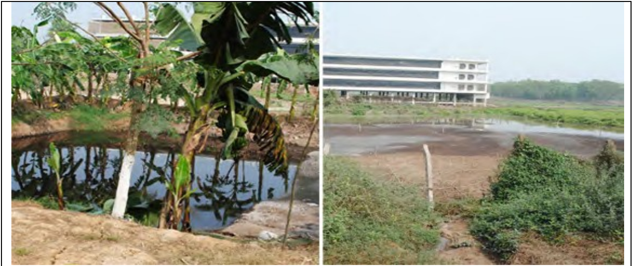
Photo 4: Slurry Drying Ponds
