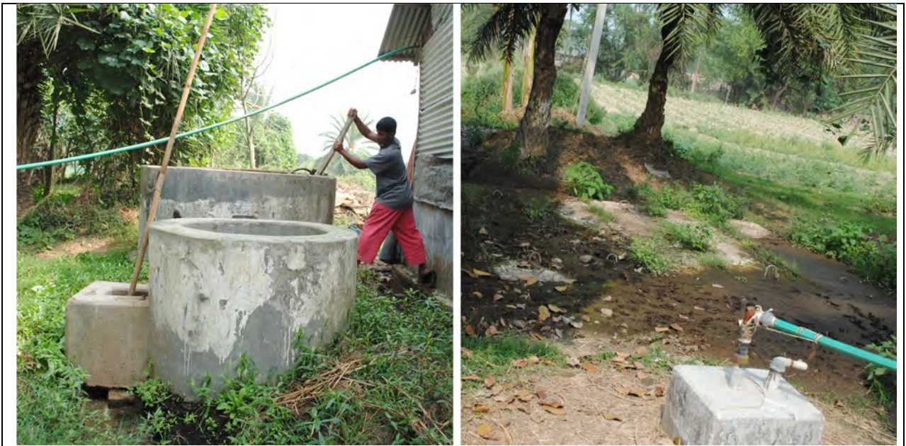
Photo 2: Biogas Plant for Cow Manure
