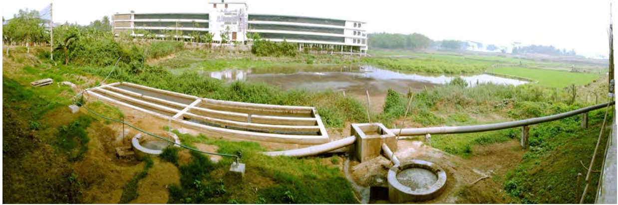
Photo 1: Biogas Plant Unit for Poultry
