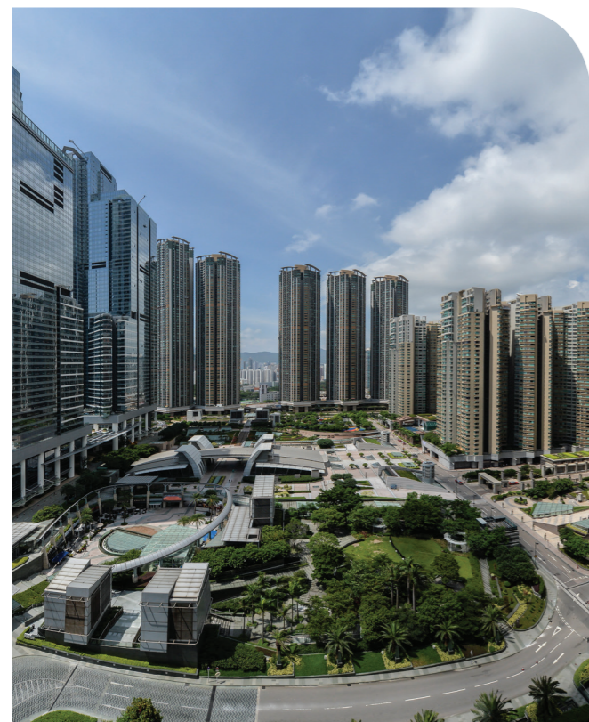
The Kowloon Station Property Development is a prominent example of MTR's Rail plus Property integrated development model.
