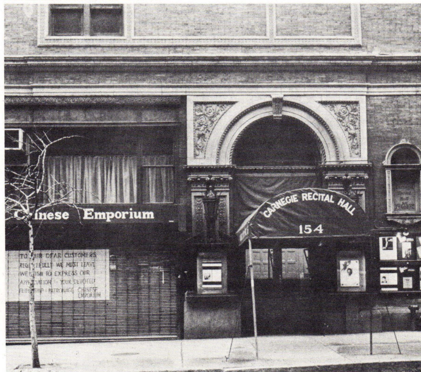
Recital Hall entrance before restoration.
