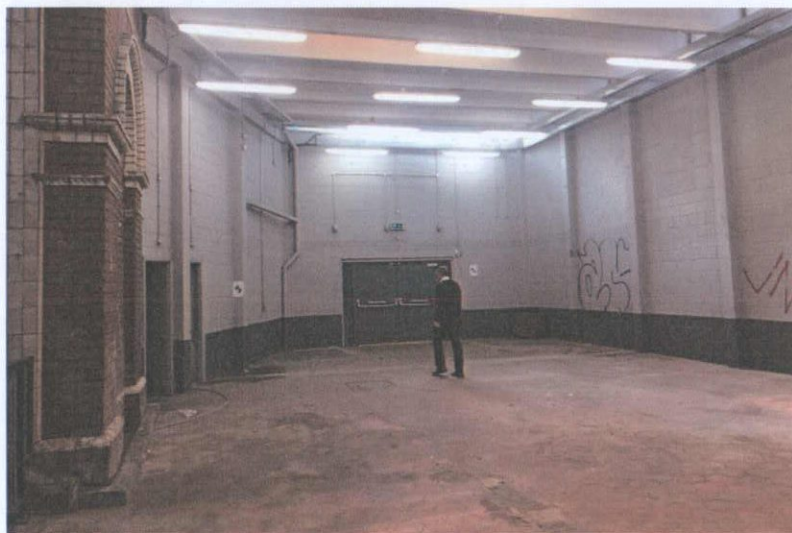
11 & 12. View of landing to steps link to DART platforms (top) and view towards entrance door in former station hall, now cleared out (bottom).
