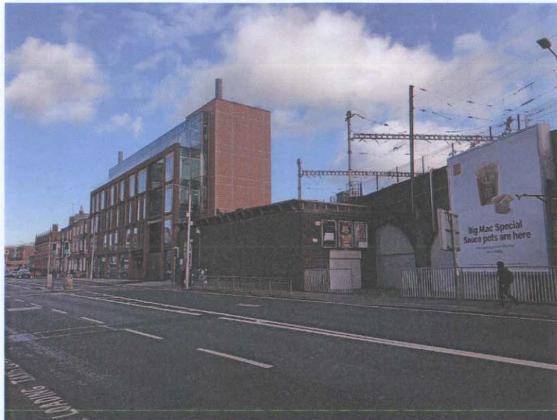
4. View along Amiens Street of former DART station hall and viaduct arches.
