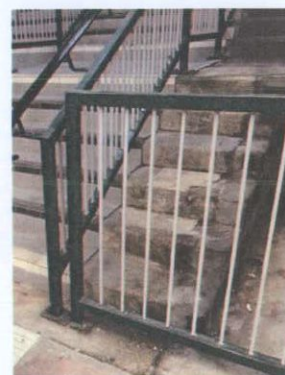
7. Detail of granite steps.
