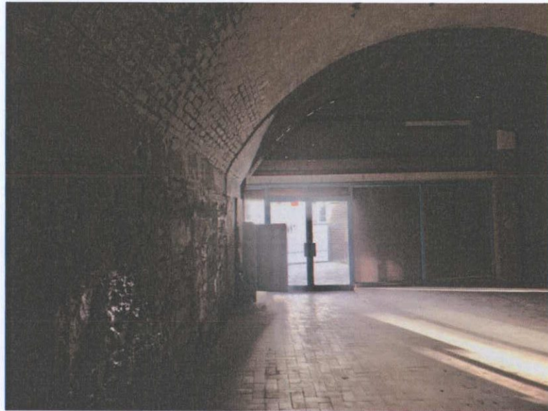
8. View of vault (former bicycle repair shop) looking towards Amiens Street.
