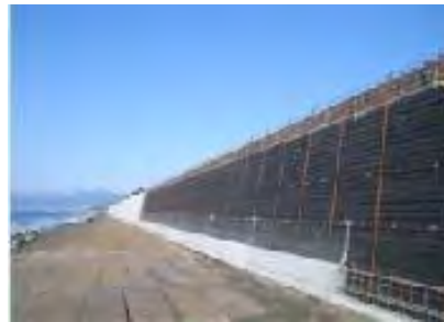
Figure: Restoration of seawall damaged by a typhoon using reinforced retaining wall
