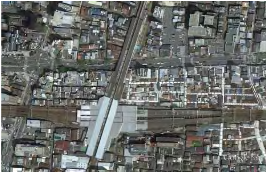
Figure 12.3-5 Example of Interconnecting Station in Japan (Tsuruhashi Station of JR West and Kintetsu)
