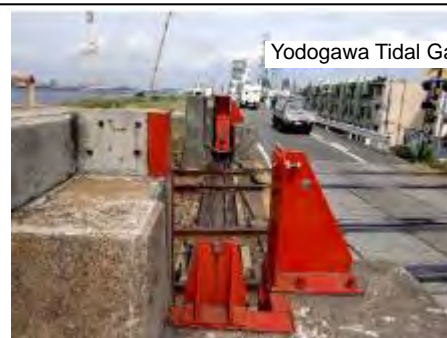
Figure: Example of a tidal gate (railway)
