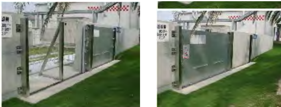
Figure: Example of cut-off wall (electrical facility)
