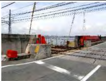
Figure: Example of a tidal gate (railway)
