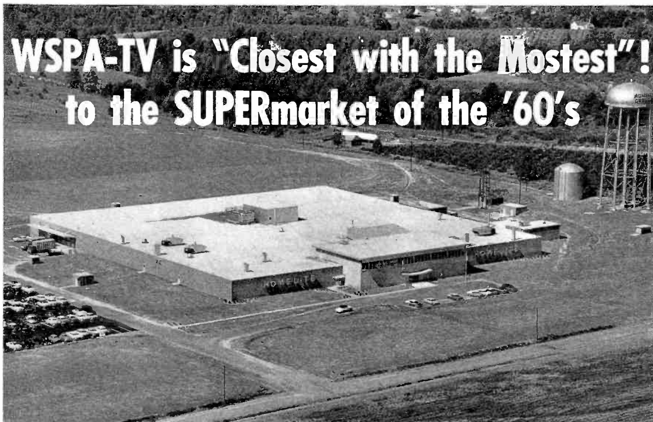
The huge new Homelite Plant at Greer, S. C.—manufacturers of chain saws, pumps and generators, employs hundreds of Carolina Piedmont area residents.
