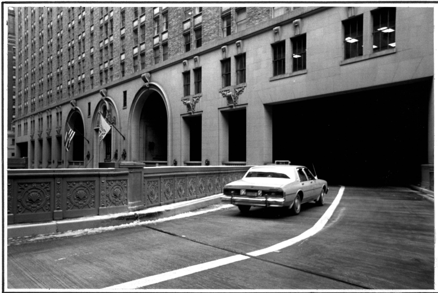
Detail: 45th Street facade from eastern viaduct
