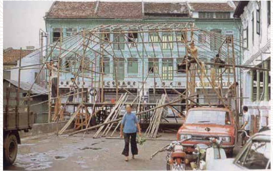
Opera stage under construction
