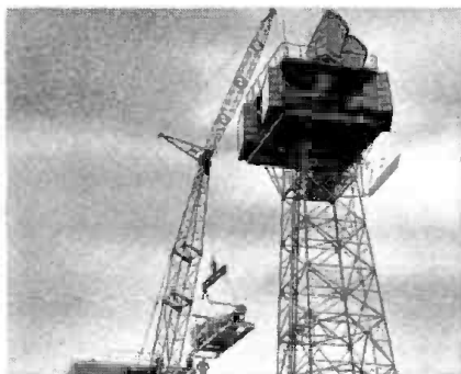
It was extending microwave routes for TV, telephone and data, and designing new facilities for future growth.
