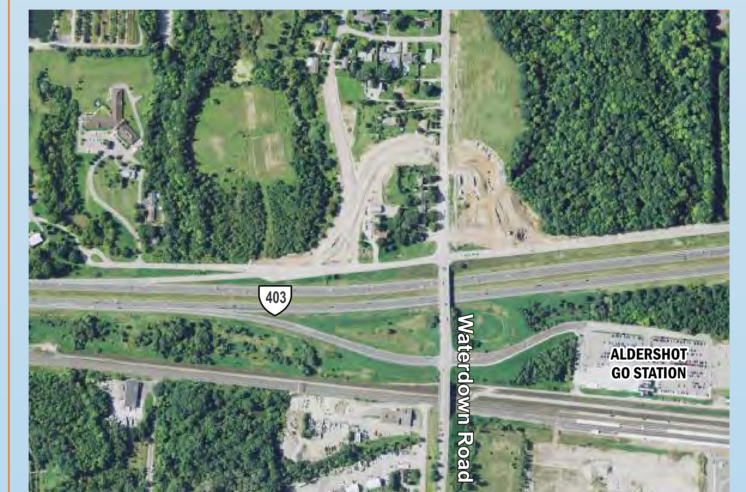
Waterdown Road Interchange expansion under construction in 2009
