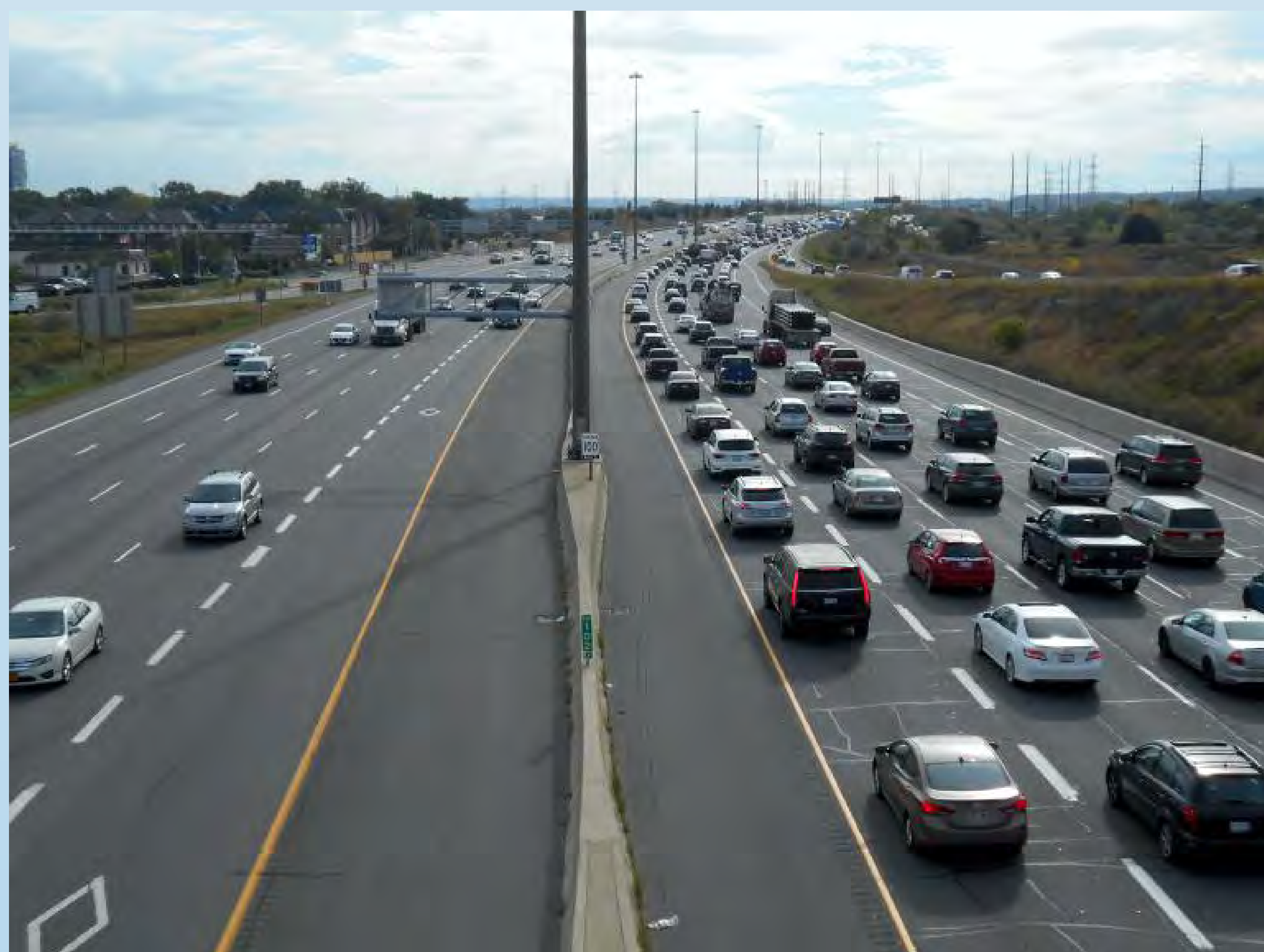
Afternoon Congestion on the Westbound QEW Approaching the Freeman Interchange
