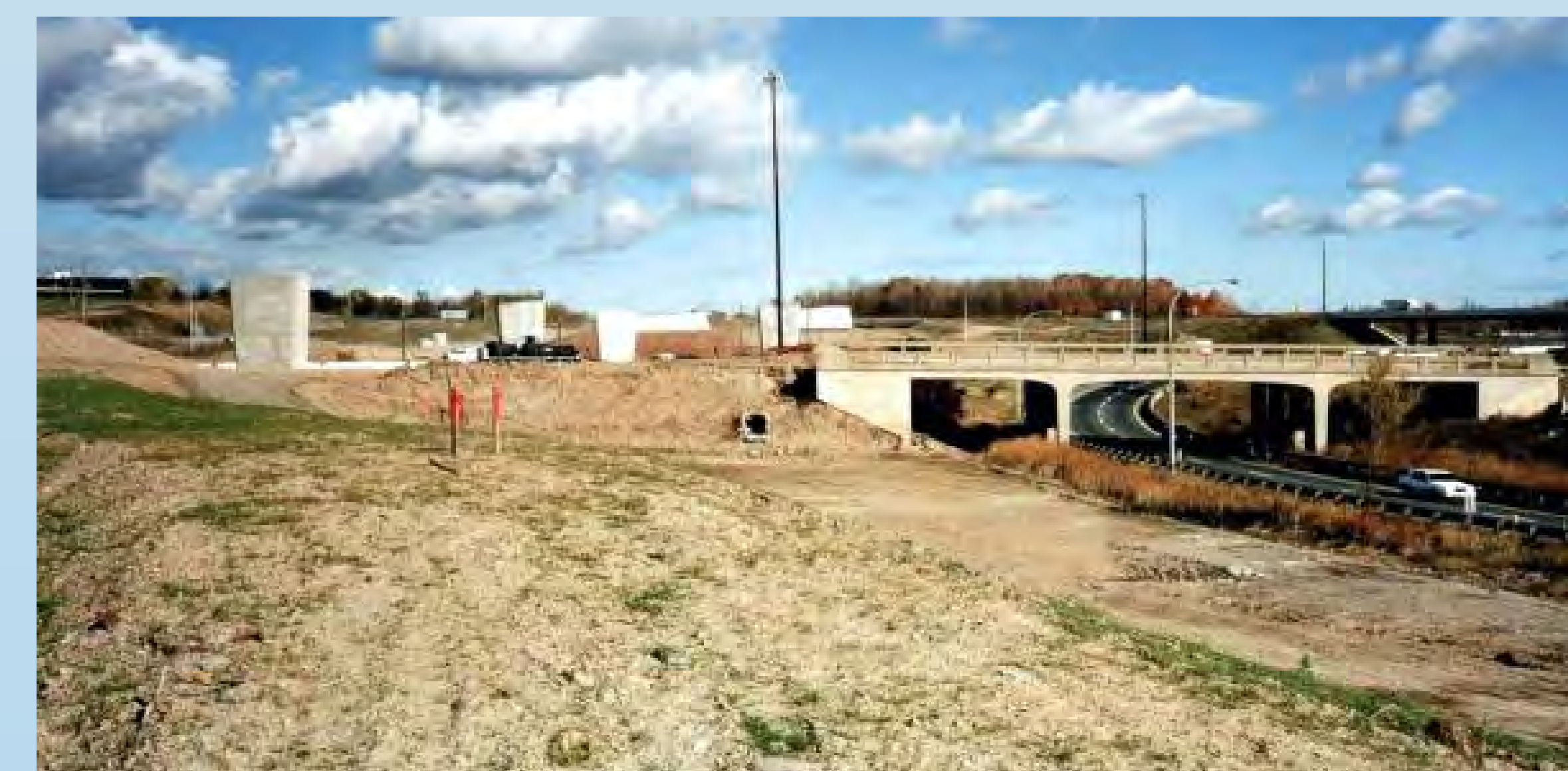
Freeman Interchange under construction in 1994
