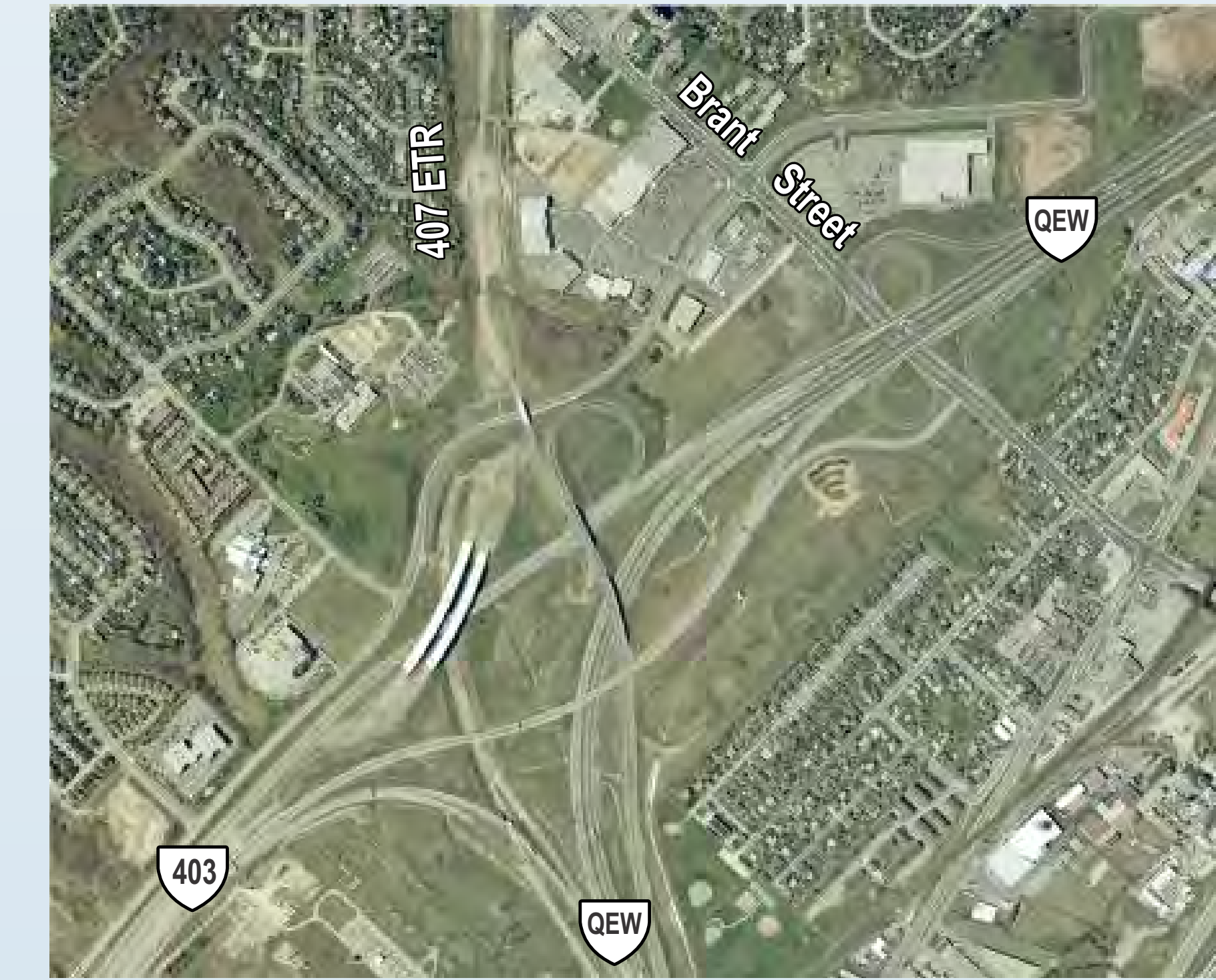
Construction of 407 ETR Connection to the Freeman Interchange
