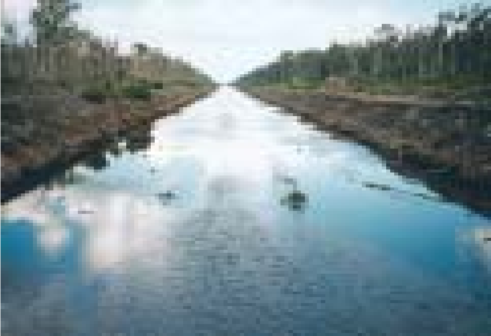
Mega Rice project drainage and irrigation channel in 1999, excavated along a tropical peatland watershed in Central Kalimantan, Indonesia. Photo: Jack Rieley & Susan Page. (§ 3.4.1 (ea))
