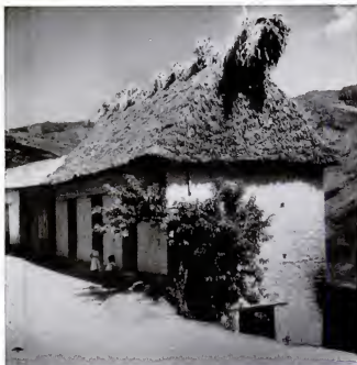
HOUSE where mushroom sessions took place is built of adobe, has thatch "dog-ears" over gable ends. Door, lower right, leads into ceremonial room.
