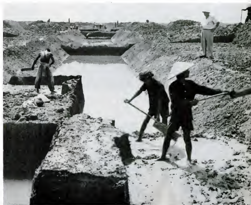
ECONOMIC DEVELOPMENT includes big reclamation projects like the Cai San Resettlement Project, where workers dig big drainage canals under direction of a U.S. technical adviser (background).
