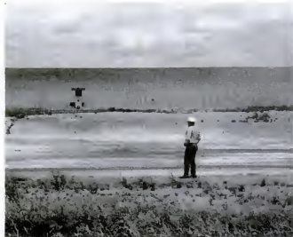
FLOOD PRECAUTION , a potential conservation pool with concrete-draw-down was built on Crews farm near Lenz, Texas during the drought. Here it is empty.
