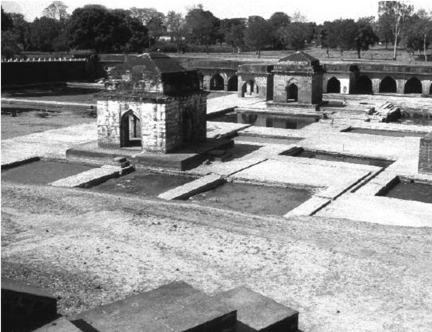
Another view of the Kalyadeh riverbed and its porticos
