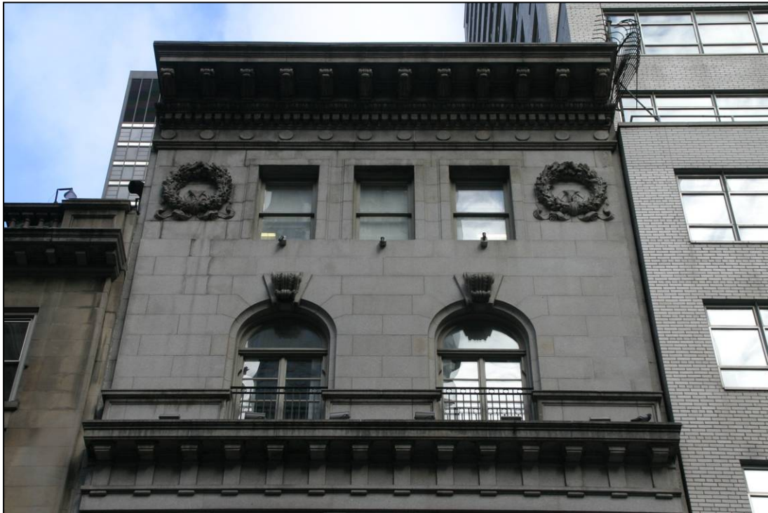
John Peirce Residence Detail of upper stories Photo: Christopher D. Brazee (2008)
