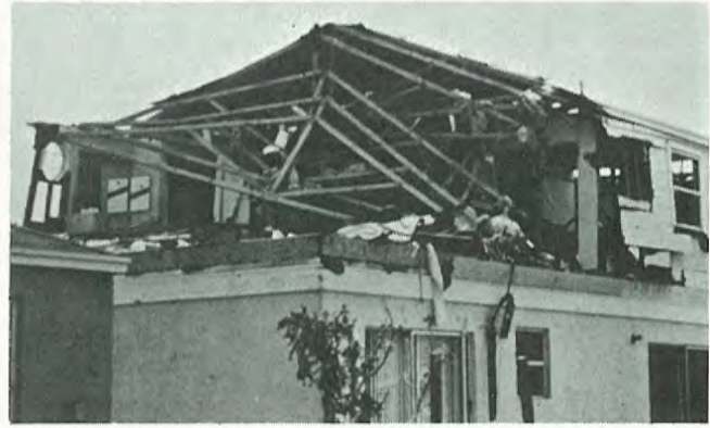
Above(left): This aerial view depicts the uneven damage pattern found in various wood structures in the Lakes By the Bay residential development. Above(right): A close-up view of a home in the development. The gable end of the roof failed during the storm. This was a frequent problem in homes of mixed wood and concrete block construction. (Photo courtesy: NHC)
