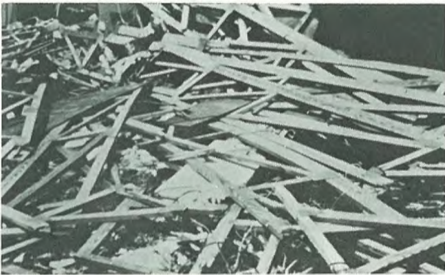
Above(left): Many roof trusses failed during the hurricane force winds. Above(right): These rustic shops were part of Gauley Square, a shopping area located north of Homestead. Both new and old buildings suffered significant damage. (Photo courtesy: NHC)
