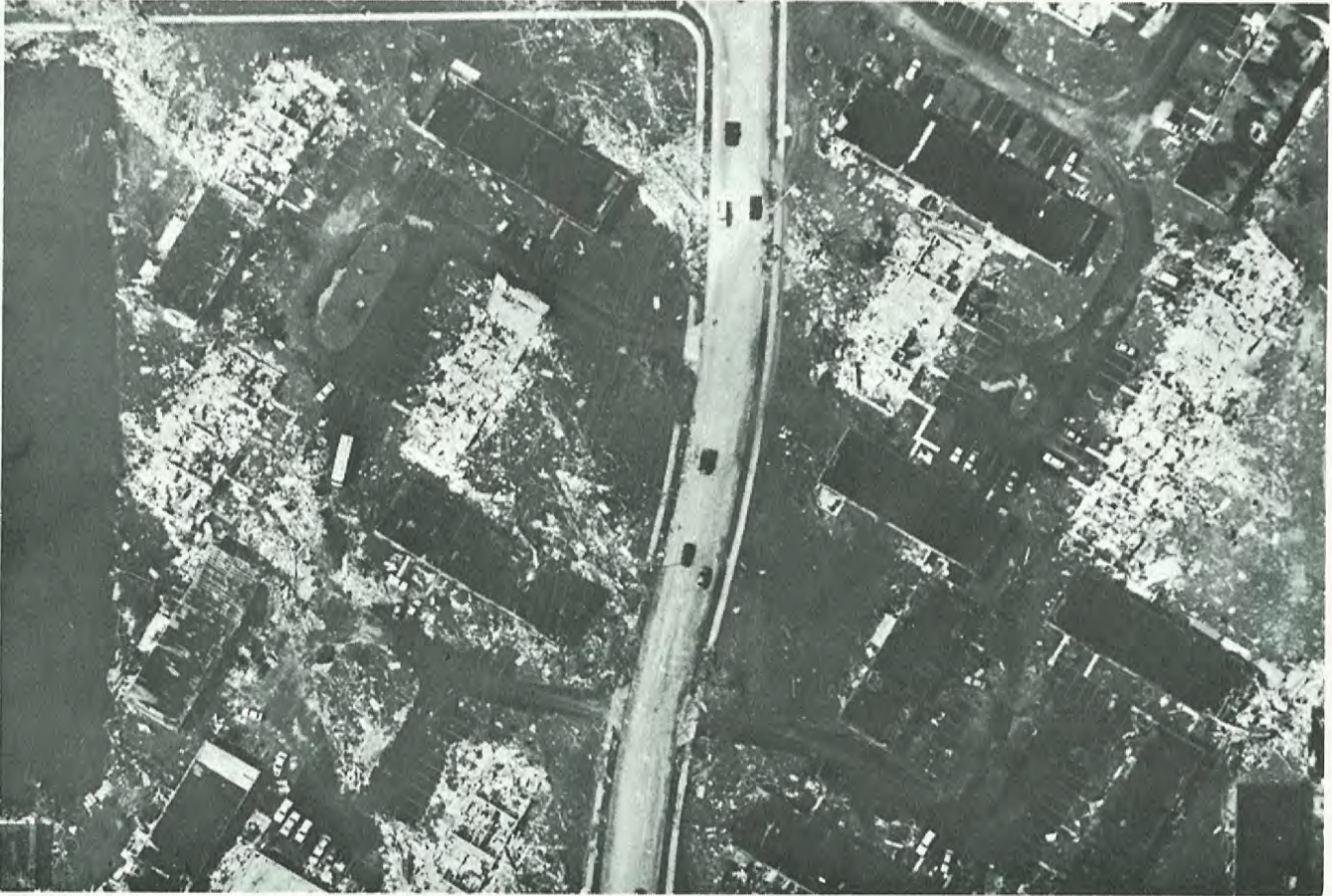
Center of Andrew's eye passed directly over Naranja Lakes, resulting in a 180^\circ shift of the first wind from NNW into the second wind from SSE. Many buildings oriented WSW-ENE (wind-perpendicular) direction received the f3 damage while those in the NNW-SSE (wind-parallel) direction were spared. Enlargement of a Continental Aerial Survey photo taken on 8/26/92.
