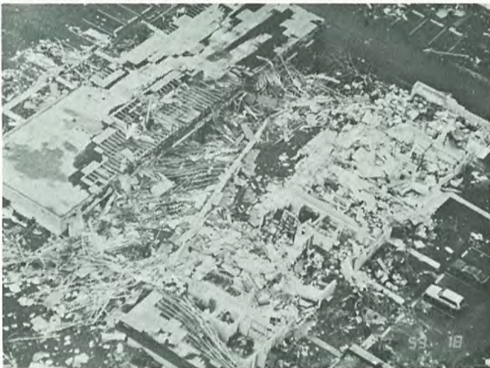
Left: A Naranja Lakes condo oriented in the wind-perpendicular (broadside) direction. The roof was lifted into a vertical position and dropped upside-down after a 180^\circ rotation. Connected and broken tie-beams weighing one ton per 20 ft are visible on the downwind side. Fujita photo 1253 EDT 9/14/92. Right: Mobile homes at Naranja Lake oriented by luck in the wind-parallel (streamline) direction. Fujita photo 0906 EDT 9/8/92.
