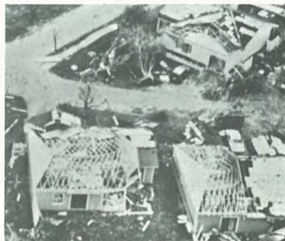
Above(left): Despite the devastation, some residents of Country Walk exhibited a sense of humor. Above(right): The roof structure of many homes in Country Walk development failed because of unsupported gables. (Photo courtesy: NHC)
