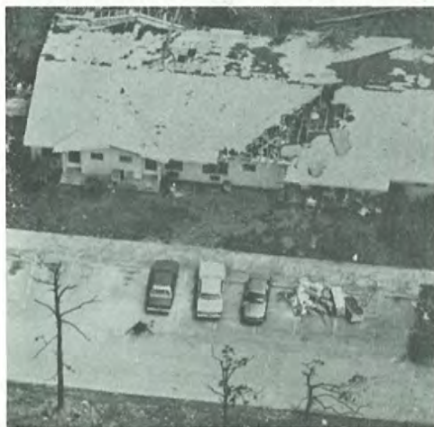
Left: An impact hole (see map) created by a falling tie-beam. Fujita photo 1245 EDT 9/14/92. A piece of flying plywood cut through the trunk of the tall pine tree shown at the lower left of the picture. Center: Drs. Robert Sheets and Peter Black examining the tree trunk. Right: A close-up view of the deep cut. Fujita photos 1057 EDT 9/9/92.
