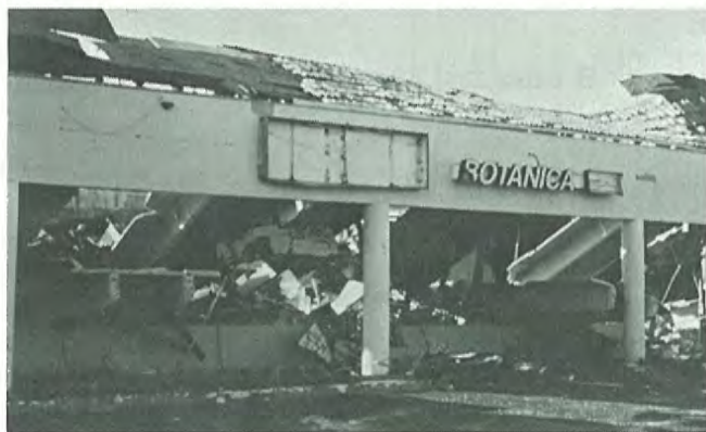
Above(left): Front view of the east (windward) face of a strip shopping center on the north side of Quail Roost Drive, near the Florida Turnpike. Winds flowing in through the broken plate glass windows, pushed the walls outward a sufficient distance to allow the pre-cast concrete roof to fall into the store. Above(right): View of the rubble inside a "Food Stop" convenience store, at the same shopping center. (Photo courtesy: Roger Edwards)
