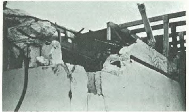
Above(left): Naranja Lakes homes were primarily concrete block and stucco (or CBS) construction. The force of Andrew's wind was strong enough to lift concrete tie beams and propel them into nearby structures. Above(right): This home in Naranja Lakes shows inadequate tie beam construction. Note that there were no vertical ties to the foundation. Many homes in Naranja Lakes lacked any vertical tie columns. (Photo courtesy: NHC)
