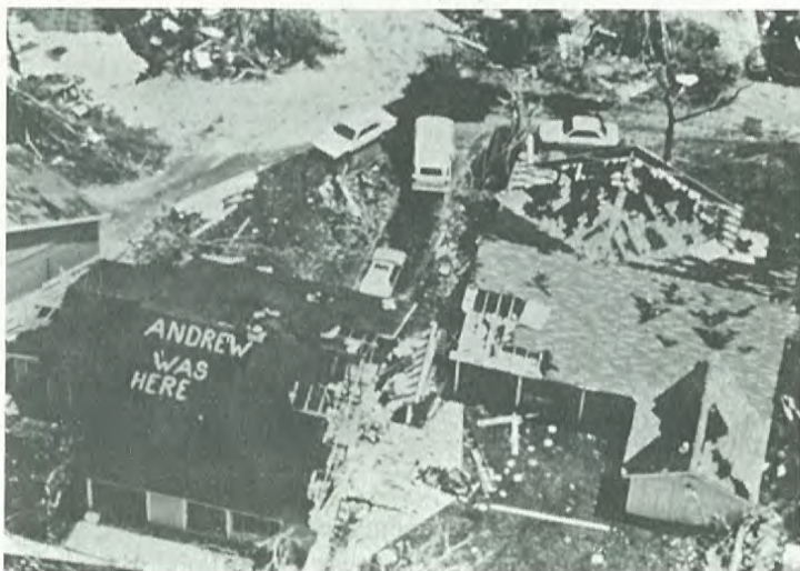
Above(left): Despite the devastation, some residents of Country Walk exhibited a sense of humor. Above(right): The roof structure of many homes in Country Walk development failed because of unsupported gables. (Photo courtesy: NHC)
