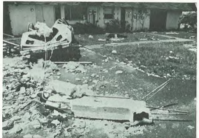
Left: An f3 damage of Naranja Lakes condo caused by a mini-swirl that formed inside the second wind. Fujita photo 1253 EDT 9/14/92. Right: Pieces of a connected tie-beam which flew 150 feet (45m) from a Naranja Lakes condo in the second wind. Fujita photo 1246 EDT 9/10/92.
