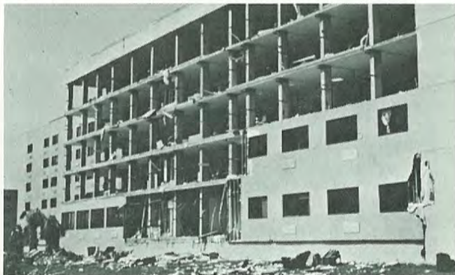
Below(right): Partial removal of the outside wall from the south (right) and west faces of the building. (Photo courtesy: Roger Edwards)
