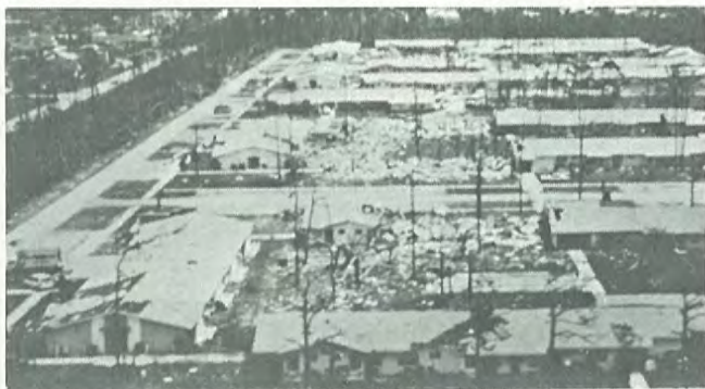
Above(left): This aerial view of a section of Pinewoods Villa, a development located in Whispering Pines, shows an uneven damage pattern. Also note the roof damage to the building located in the center foreground. This damage resulted from a tie beam that was torn from a home 300 feet away and then dropped through the roof of the structure. Above(right): A view of the tie beam from inside the structure. This type of tie beam typically weighs at least 1,000 pounds! (Photo courtesy: NHC)
