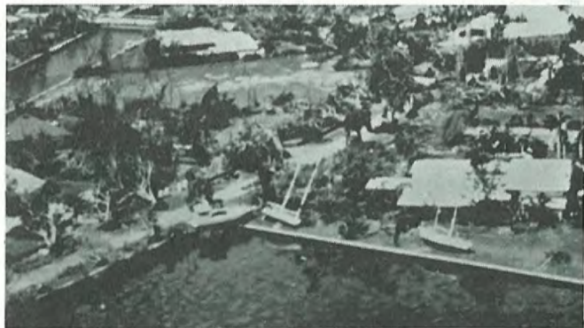
Above(left): Sewell Park before Andrew. Above(right): Sewell Park early morning of August 24. Below: The Gables-by-the-Sea marina located near Gables Estates where numerous boats were forced ashore by the 9 to 16 foot storm surge. Also note the downed trees. (Photo courtesy: NHC)
