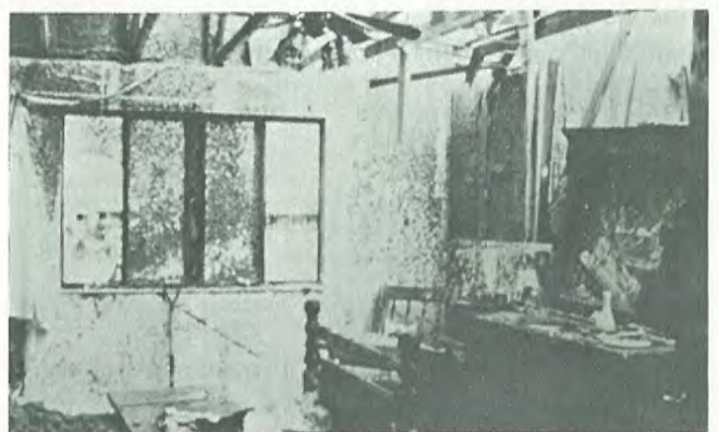
Above(left): The frame is all that remains of this mobile home. This demonstrates the high risk to residents who must ride out severe wind storms in such a structure. Above(right): A damaged home in the Saga Bay development clearly shows the damage inflicted by high wind and heavy rain. Insulation is splattered across the bedroom walls. (Photo courtesy: NHC)
