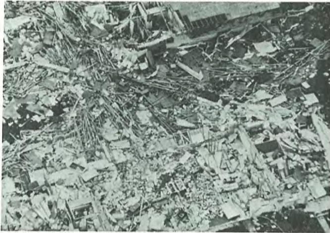
Left: An f3 damage of Naranja Lakes condo caused by a mini-swirl that formed inside the second wind. Fujita photo 1253 EDT 9/14/92. Right: Pieces of a connected tie-beam which flew 150 feet (45m) from a Naranja Lakes condo in the second wind. Fujita photo 1246 EDT 9/10/92.
