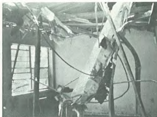
Above(left): This aerial view of a section of Pinewoods Villa, a development located in Whispering Pines, shows an uneven damage pattern. Also note the roof damage to the building located in the center foreground. This damage resulted from a tie beam that was torn from a home 300 feet away and then dropped through the roof of the structure. Above(right): A view of the tie beam from inside the structure. This type of tie beam typically weighs at least 1,000 pounds! (Photo courtesy: NHC)
