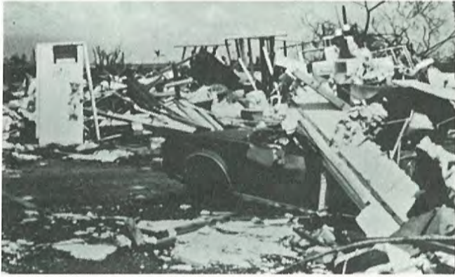
Above(left): Naranja Lakes homes were primarily concrete block and stucco (or CBS) construction. The force of Andrew's wind was strong enough to lift concrete tie beams and propel them into nearby structures. Above(right): This home in Naranja Lakes shows inadequate tie beam construction. Note that there were no vertical ties to the foundation. Many homes in Naranja Lakes lacked any vertical tie columns. (Photo courtesy: NHC)
