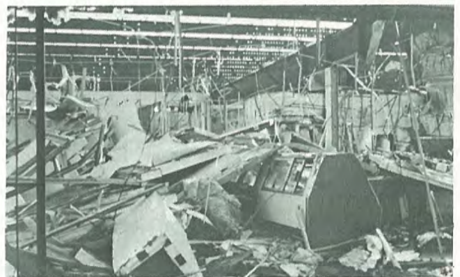
Above(left): Front view of the east (windward) face of a strip shopping center on the north side of Quail Roost Drive, near the Florida Turnpike. Winds flowing in through the broken plate glass windows, pushed the walls outward a sufficient distance to allow the pre-cast concrete roof to fall into the store. Above(right): View of the rubble inside a "Food Stop" convenience store, at the same shopping center. (Photo courtesy: Roger Edwards)
