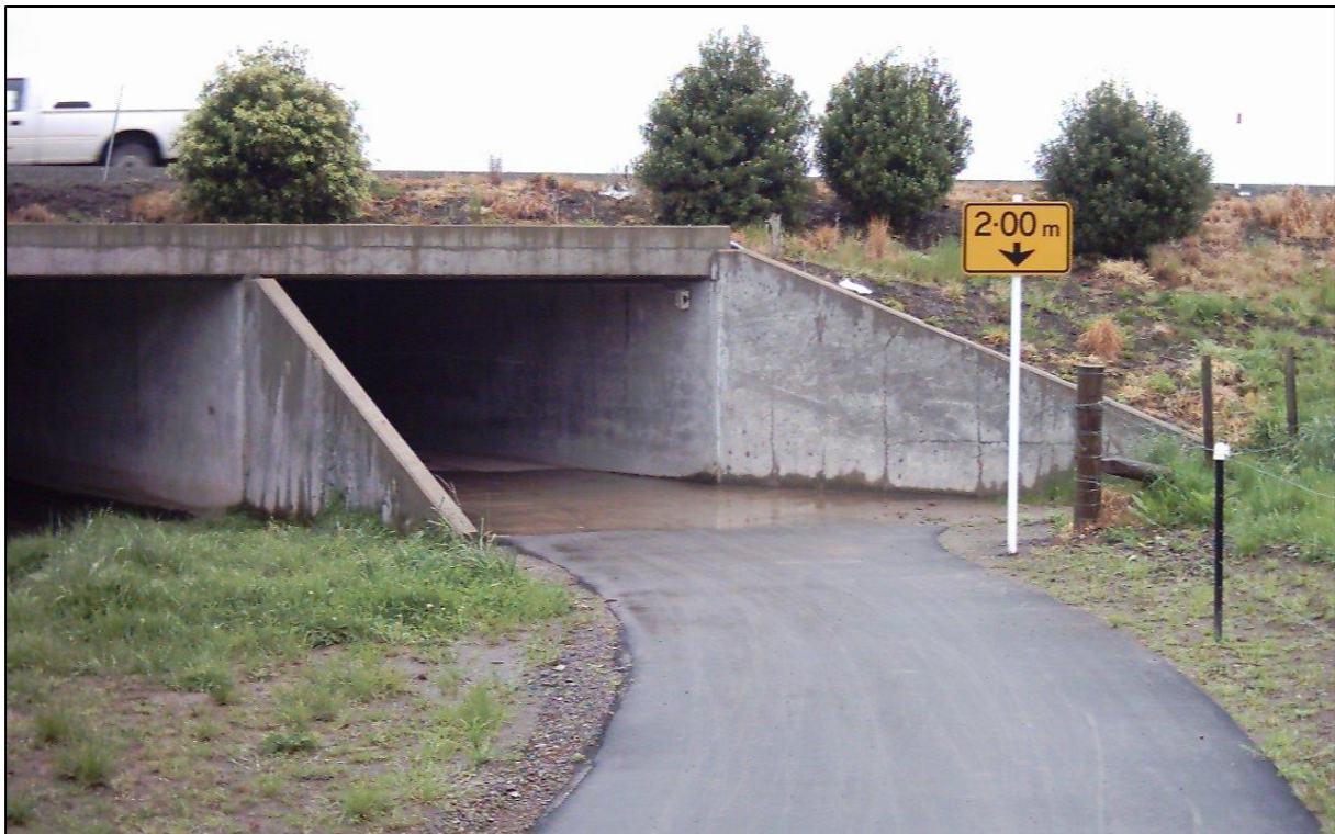
Figure 21: Warning sign for a low underpass, Nelson
