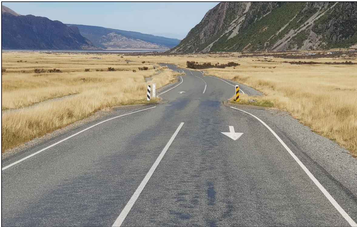
Figure 42: An example of rural traffic calming on a 60 km/h road, Hooker Valley
