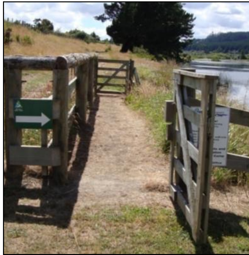
Figure 75: Double gate, Waikato River Trail
