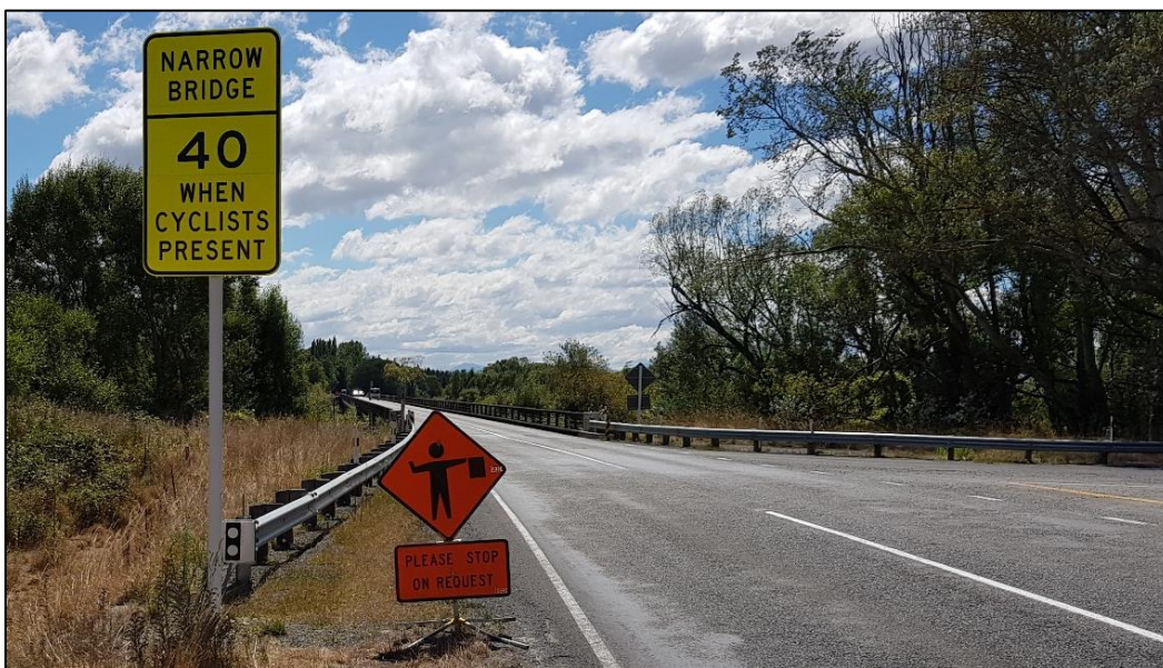
Figure 55: Example of an advisory speed sign on a narrow State Highway bridge, Hurunui
