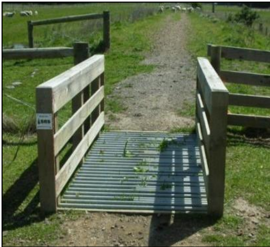
Figure 69: Cattle stop placed on straight alignment of track
