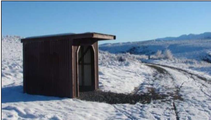
Figure 102: Shelter on Otago Central Rail Trail (photo: DOC)
