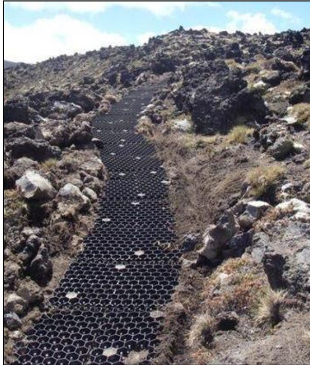
Figure 27: "Geomat" surface stabilisers (prior to having aggregate placed on top), Tongariro National Park (photo: John Bradley)
