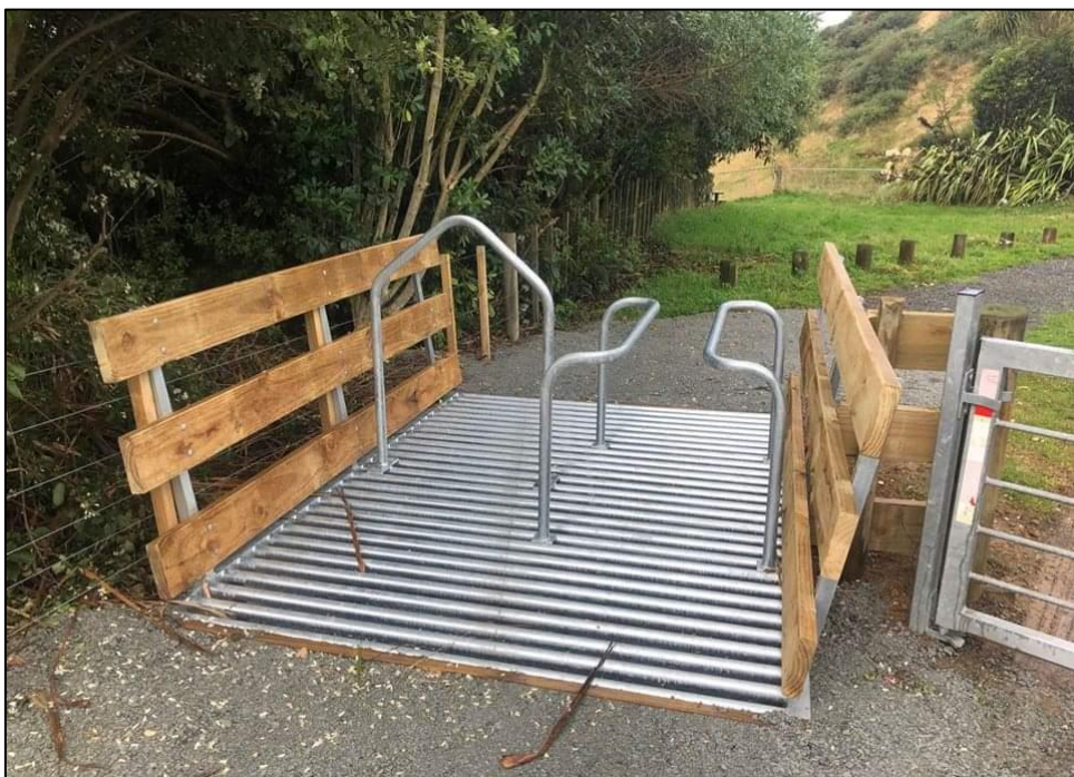
Figure 34: Example of a wheelchair-accessible barrier, Belmont Regional Park (photo: Greater Wellington Regional Council)
