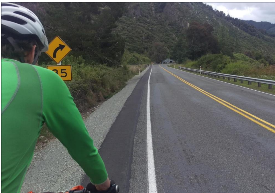
Figure 49: Smooth shoulder widening, SH6 near Murchison (photo: Miro Kennett)
