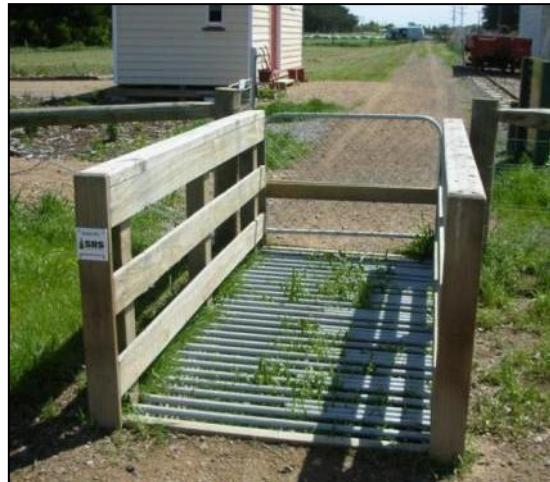
Figure 70: Gate added – a poor solution for cycling
