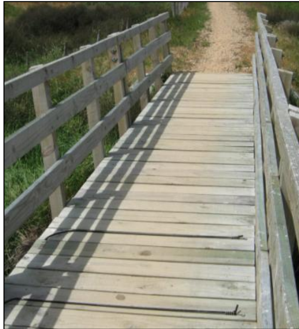
Figure 107: Pneumatic tubes installed on off-road trail bridge
