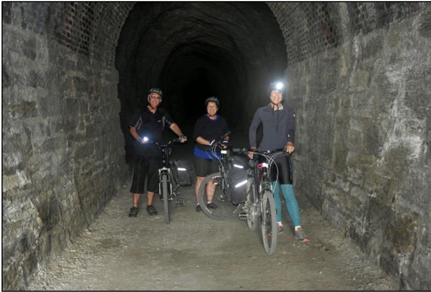
Figure 104: Cyclists with headlamps in tunnel on Otago Central Rail Trail
