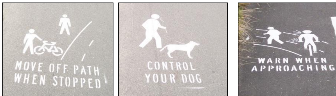
Figure 33: Shared path markings, Nelson
