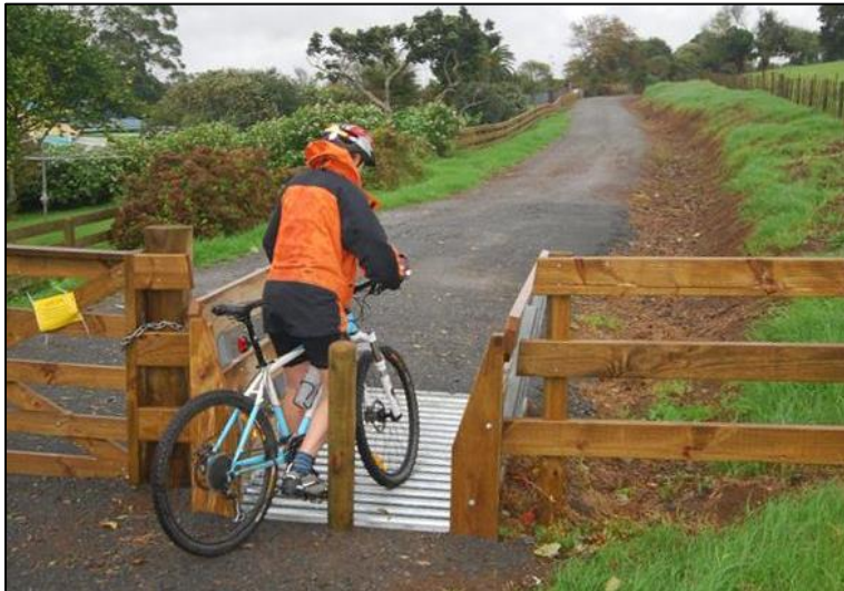
Figure 73: A central post and wing barriers help prevent motor-cycle access and reduce the likelihood of stock jumping the cattle stop, but also led to complaints from cyclists with panniers (photo Jonathan Kennett)
