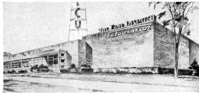
WICU (TV) building now under construction.
