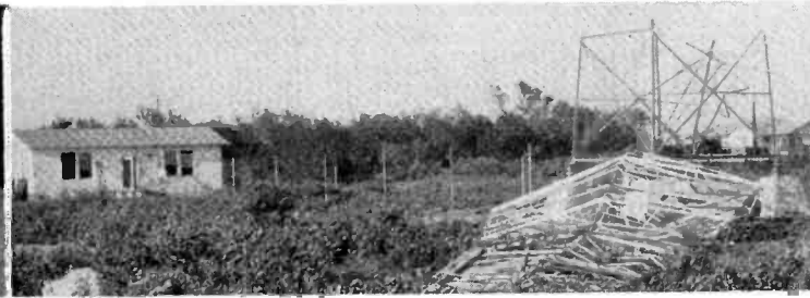
SNAPPED off almost to the base, the 152-foot self-supporting steel tower of WKWF Key West lies sprawled on the ground, blown over by the recent hurricane that roared over the Keys. Only 20 minutes after the tower collapsed, the station was back on the air with an emergency antenna.
