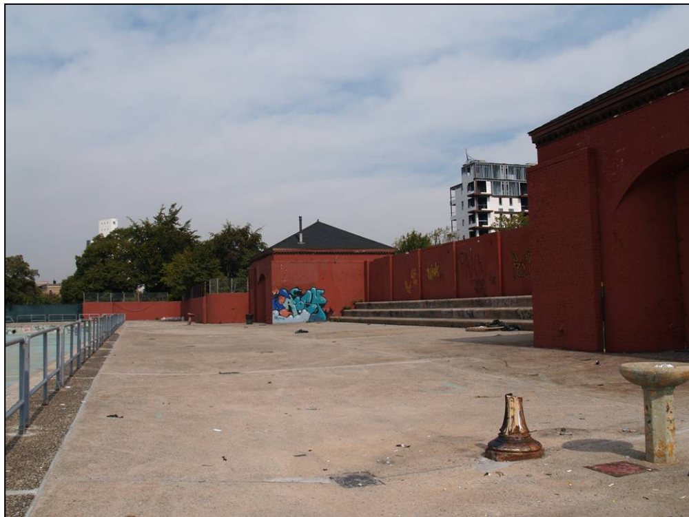
McCarren Play Center filter house: view looking northeast. Photo: Zerina Philip, NYC Parks Dept., 2006
