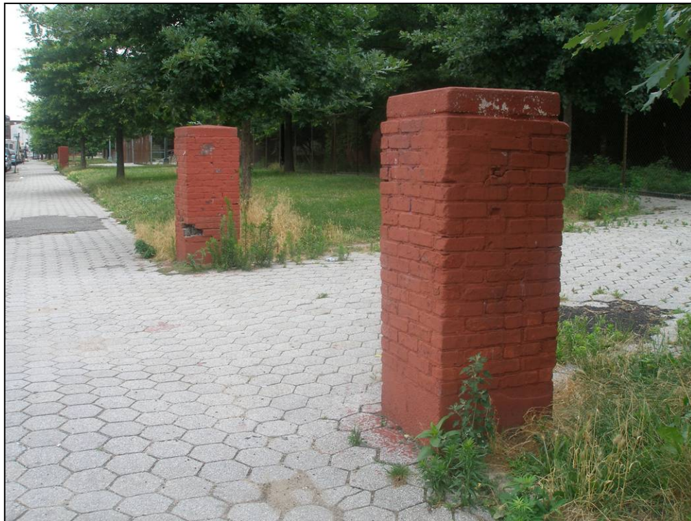
McCarren Play Center: remnants of perimeter walls. Looking north, from corner of Lorimer and Bayard.
