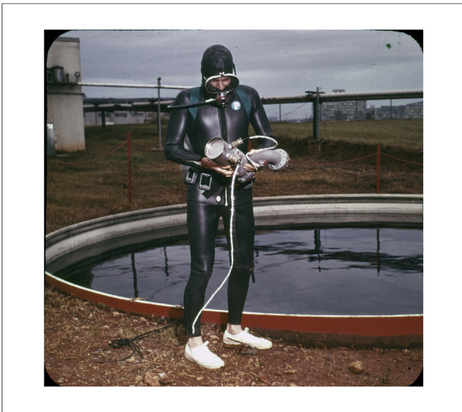
Figure 4. A diver, likely Charlie Cooper, holding a S-IVB propellant utilization valve at NASA Marshall Space Flight Center's 8-foot explosive-forming tank, November 1965.
