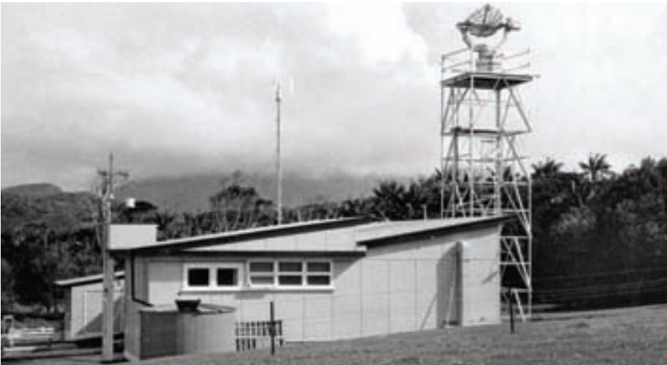
WWII Royal Navy radar turned weather radar, Lord Howe Island field office, 1958.
