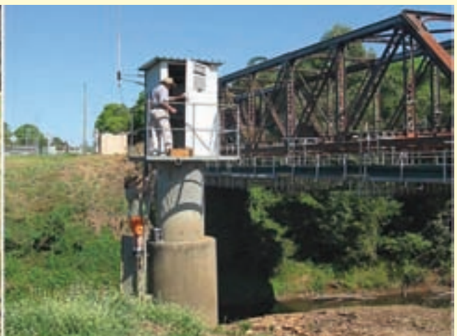
Maintenance on an automatic river height gauge on Wilsons River near Lismore.
