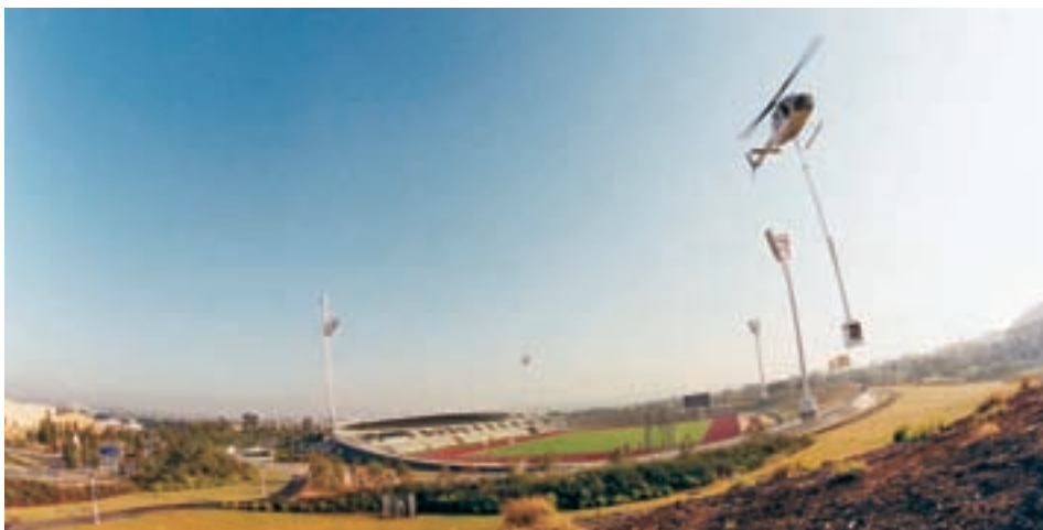
Lowering an automatic weather station on to the Homebush site, 2000 Sydney Olympics.
