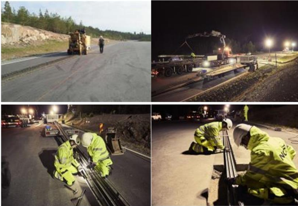
Figure B.14: Elways Installation Process (Source: Elways)
