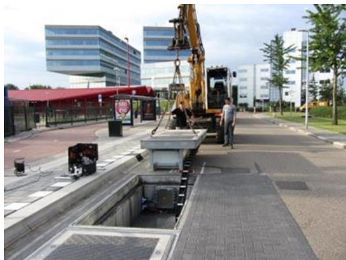
Figure B.9: IPT Installation (Source: IPT Technologies)
