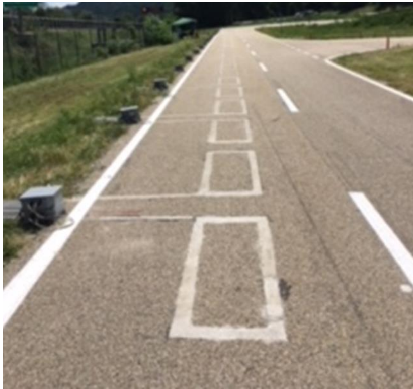
Figure B.4: CWD Installation
