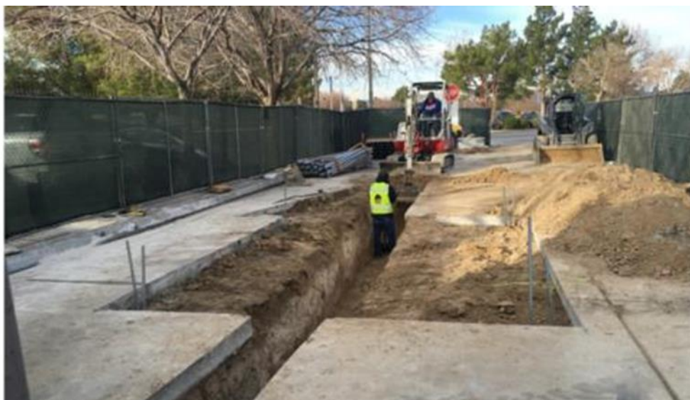
Figure B.18: WAVE IPT Installation (Source: Wave IPT)
