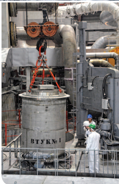
Construction stage, July 2011 ▲ Installation of the on-site transportation package set in the reactor hall ◀
