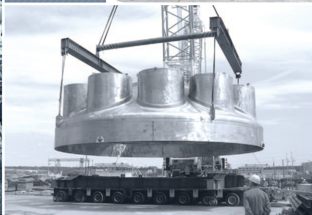
Installation of the reactor head ▲▼ Construction stage, June 2009 ◀
