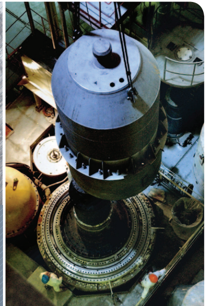
Installation of the BN-600 vessel
