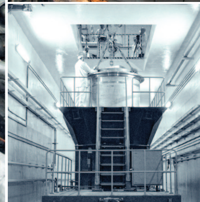
Construction stage, July 2011 ▲ Installation of the pump ▶
