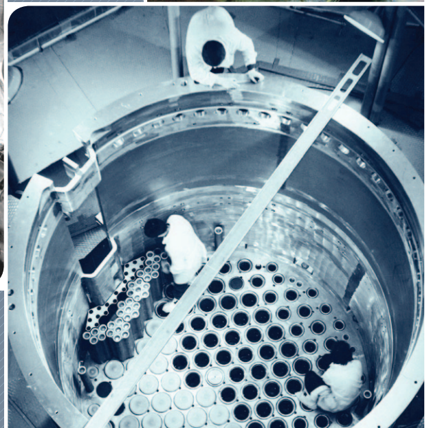
Installation of the BN-600 large rotating plug ▲
