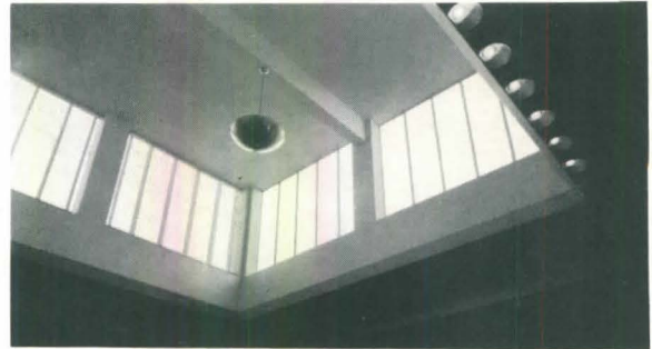
Fig. 6 CLERISTORY WINDOWS throw high side light on the object without throwing it into the eyes of the spectator. Same result is achieved at night by appropriate arrangement of artificial light
