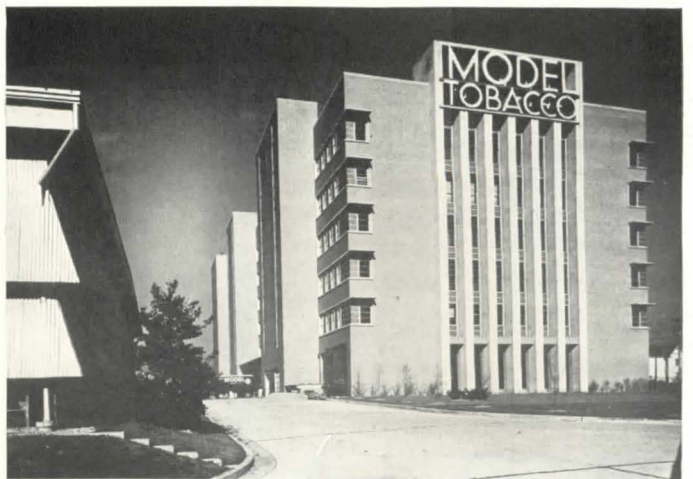
TRUCKING LANE (warehouse at left)
