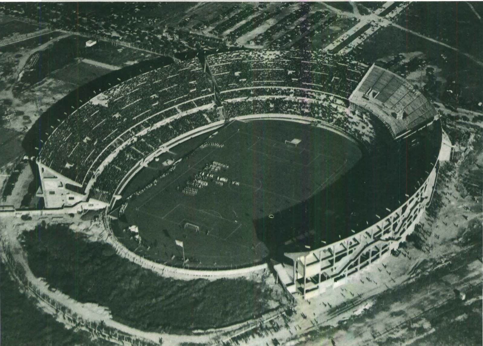
CIRCULAR STADIUM; RIVER PLATE CLUB, BUENOS AIRES, ARGENTINA: JOSE ASLAN, HECTOR EZCURRA, ARCHITECTS
