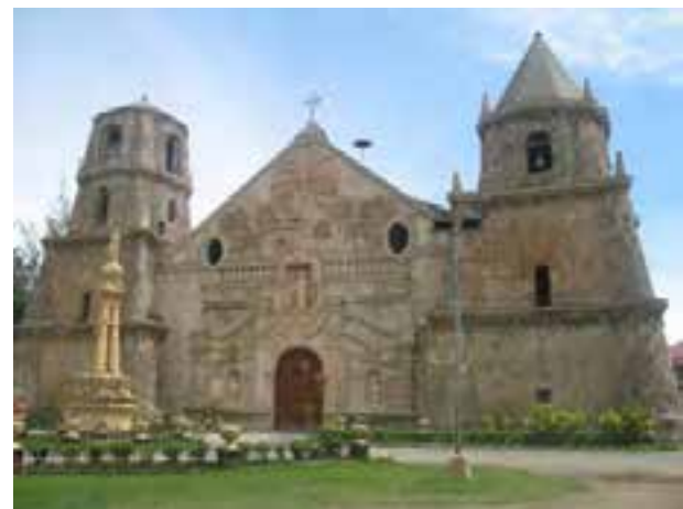
The Cleaning and Restoration of exterior masonry walls of Miagao Church in Miagao, Iloilo was completed in February 2010. The project was funded by NCCA and implemented by the National Museum.
