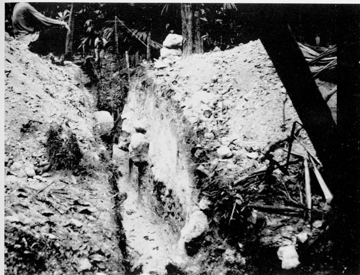
Looking north through the excavation of the embankment shown in Fig. 2. Note the dark color of the original topsoil level beneath the embankment.
