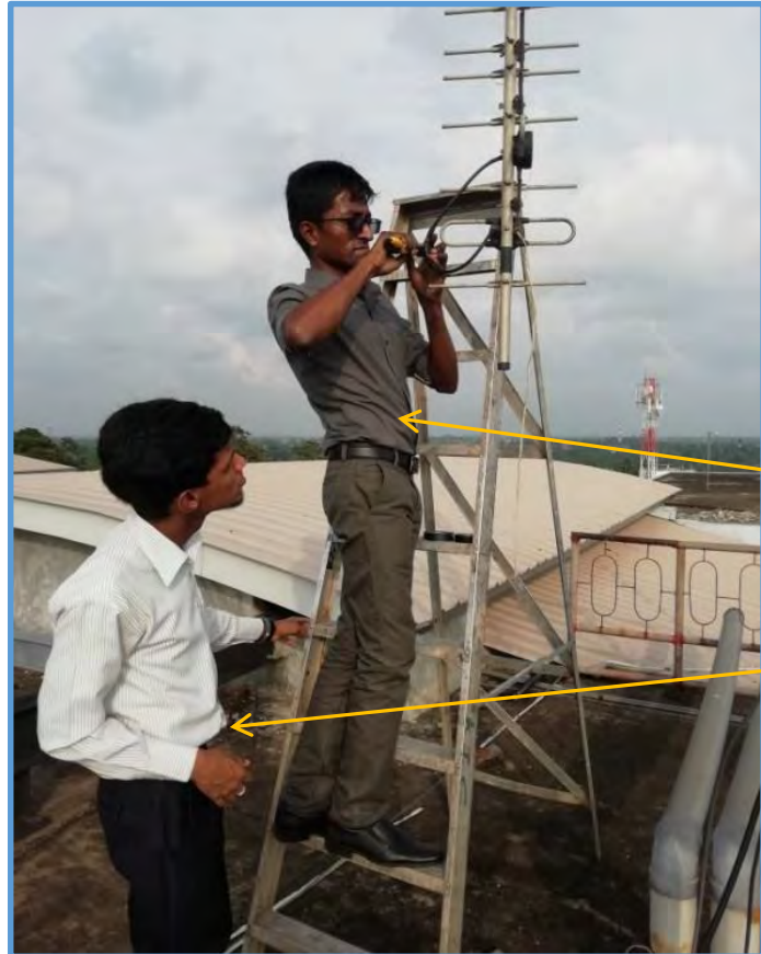
UHF Antenna maintenance and Connector fixing
