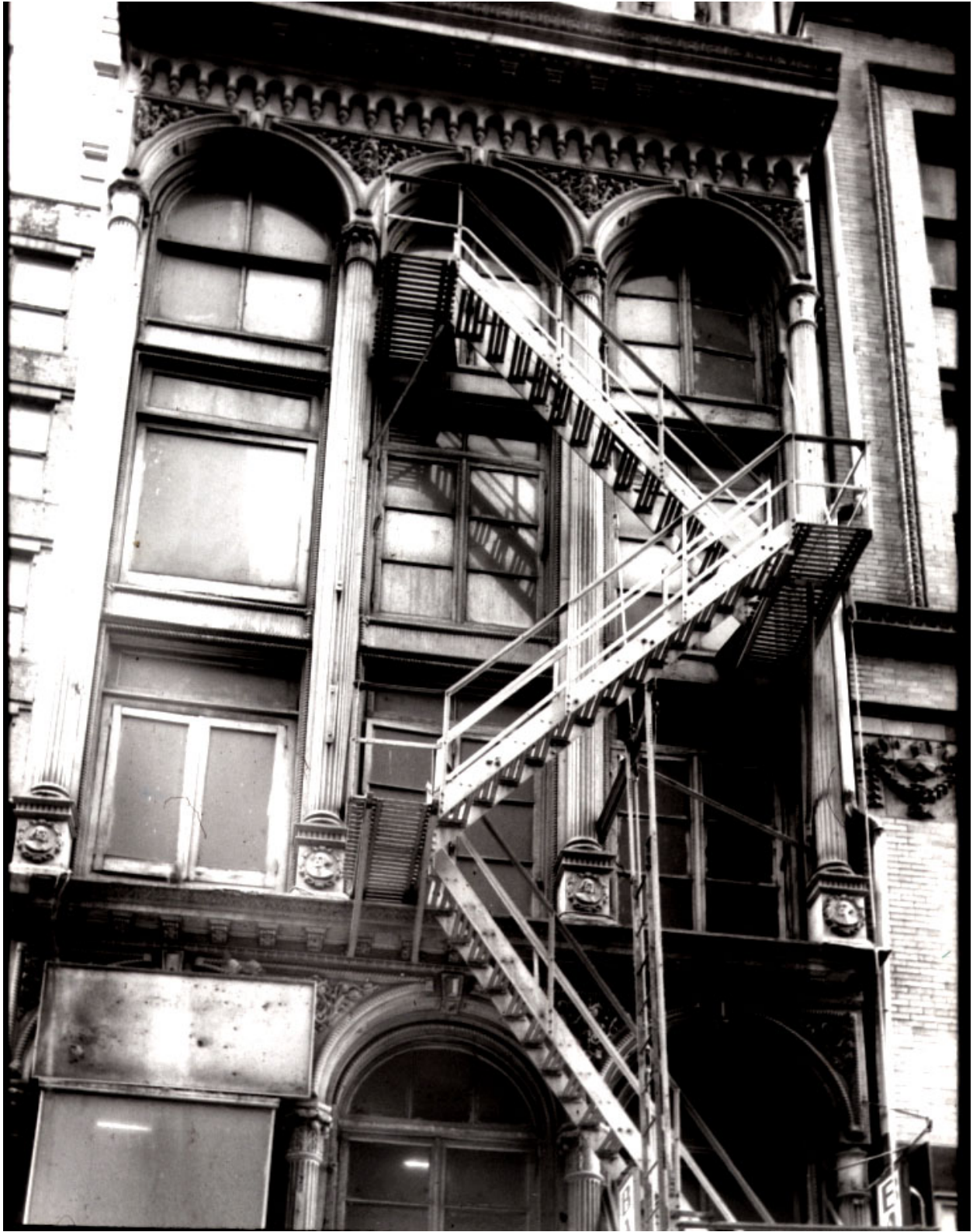
63 Nassau Street Building , Manhattan
