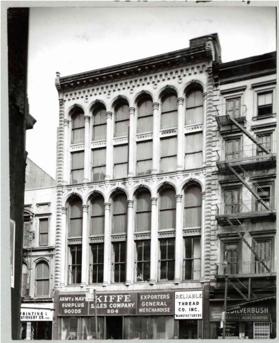
502-504 Broadway (1860, John Kellum & Son), masonry façade
