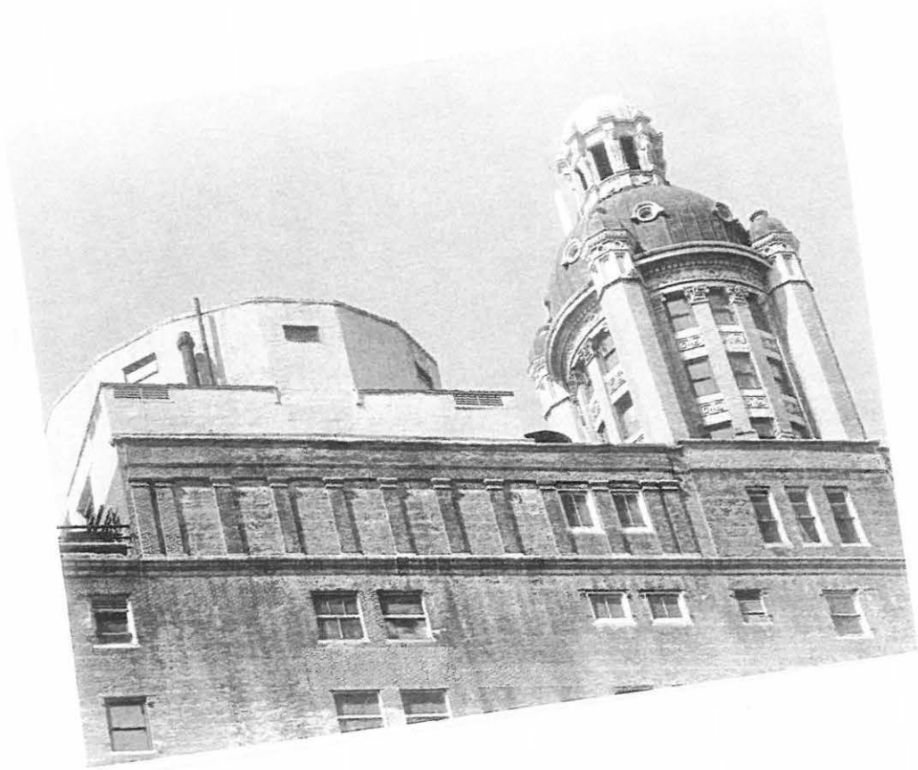
Park Row Building roof-top addition, north tower Photo: Carl Forster
