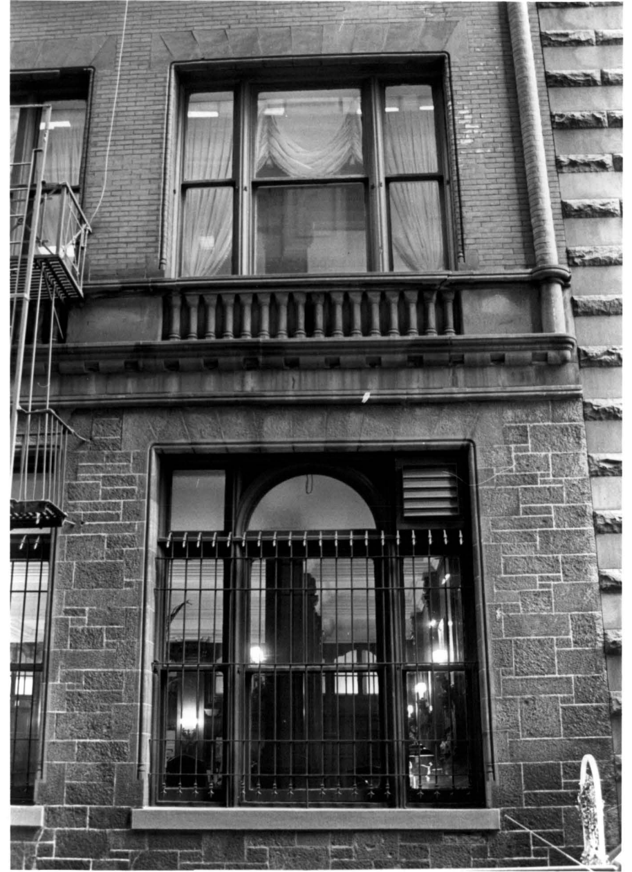
The Down Town Association Building, window details, Cedar Street facade
