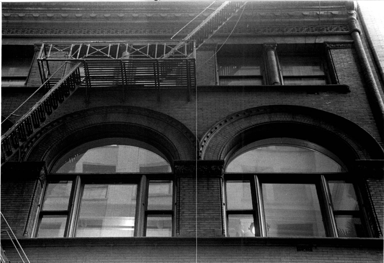
The Down Town Association Building, window detail, Cedar Street facade
