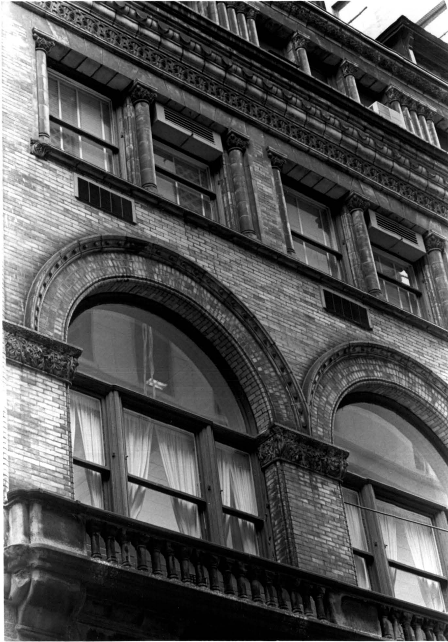
The Down Town Association Building, window details, Pine Street facade
