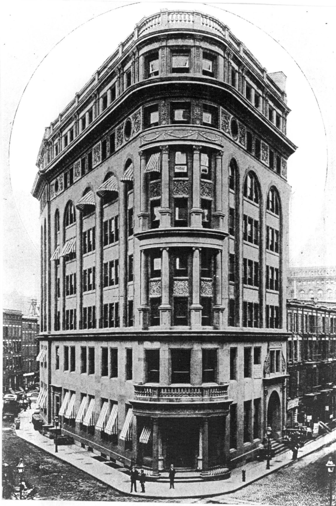
View of the Delmonico Building, c. 1891
