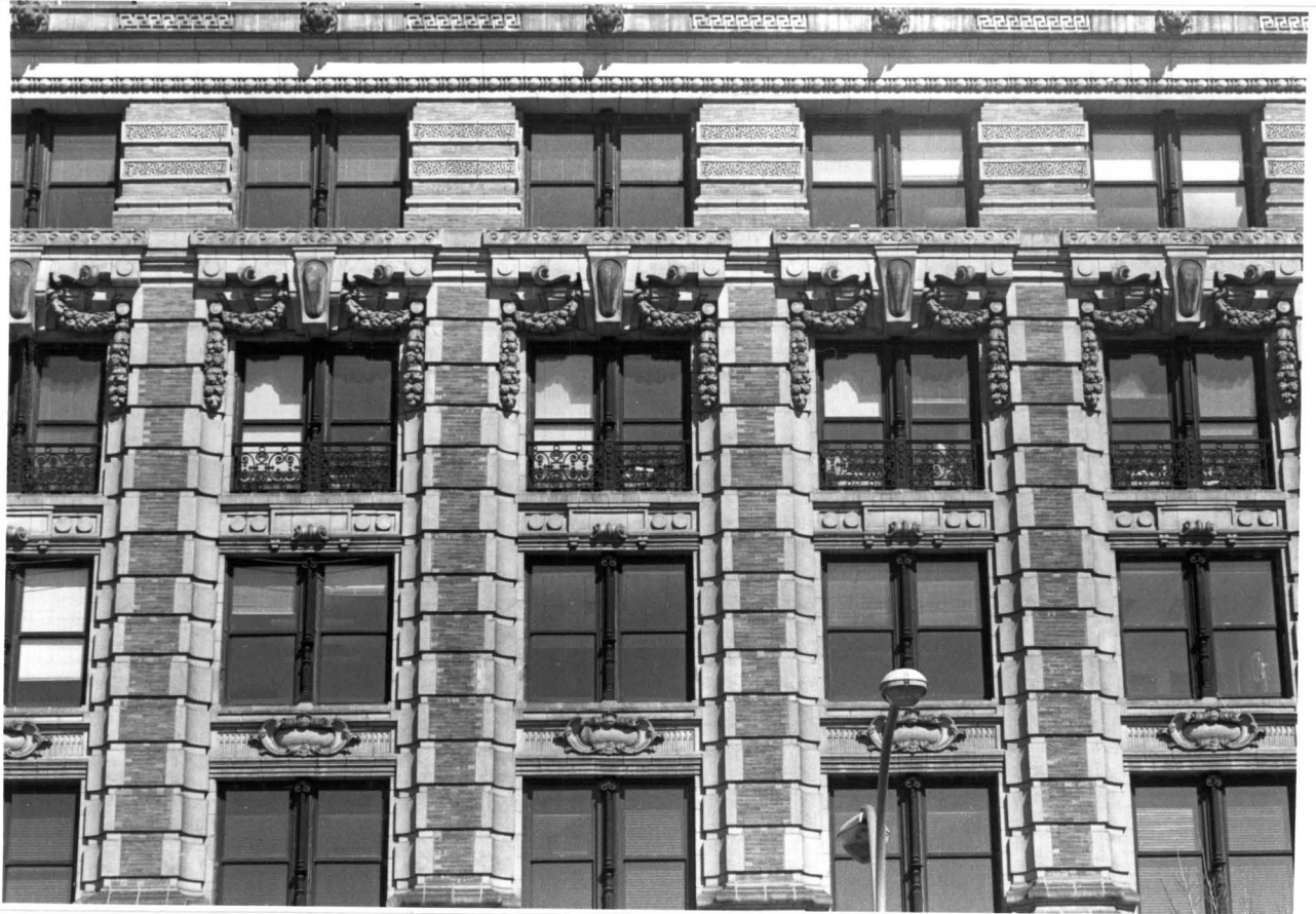
The Whitehall Building Details, Battery Place facade Photo: Carl Forster
