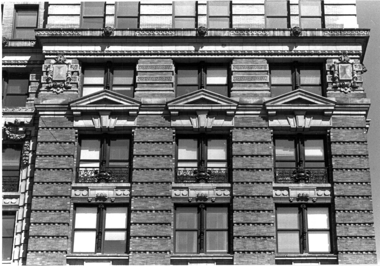
The Whitehall Building Window details, Battery Place facade Photos: Carl Forster
