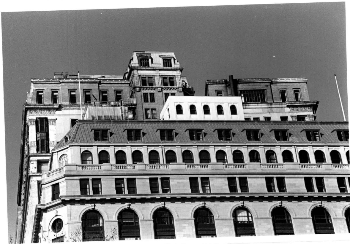
Fig. 16 Bowling Green Offices, South elevation (part of No. 1 Broadway in foreground) Photos: DMB
