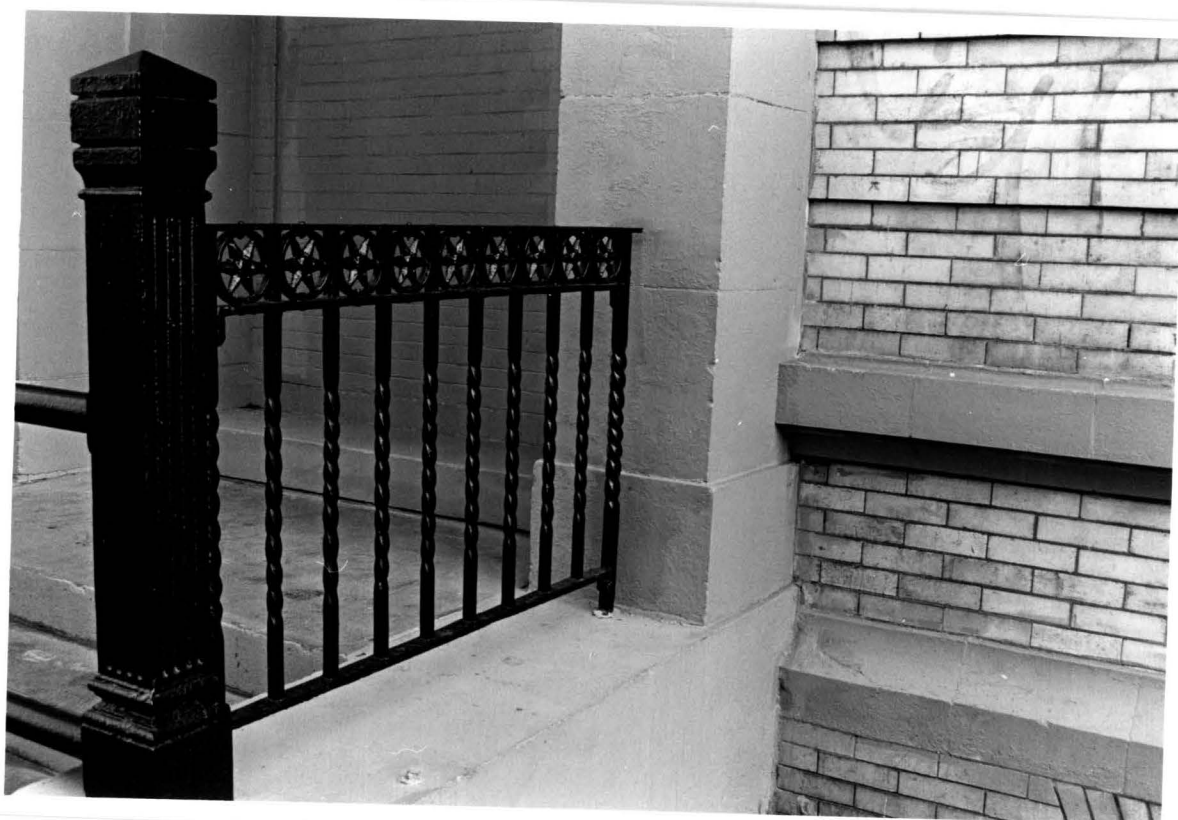
Fig. 15 Bowling Green Offices, Detail of ironwork on Greenwich Street
