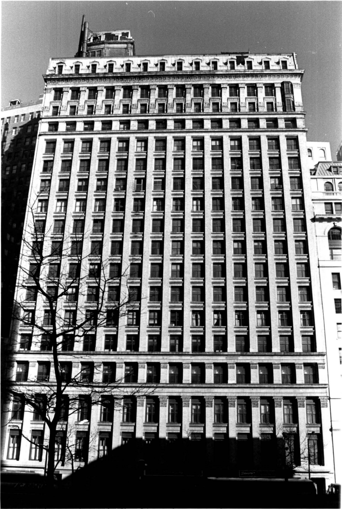
Fig. 11 Bowling Green Offices Building, 5-11 Broadway, Greenwich Street facade Photo: DMB
