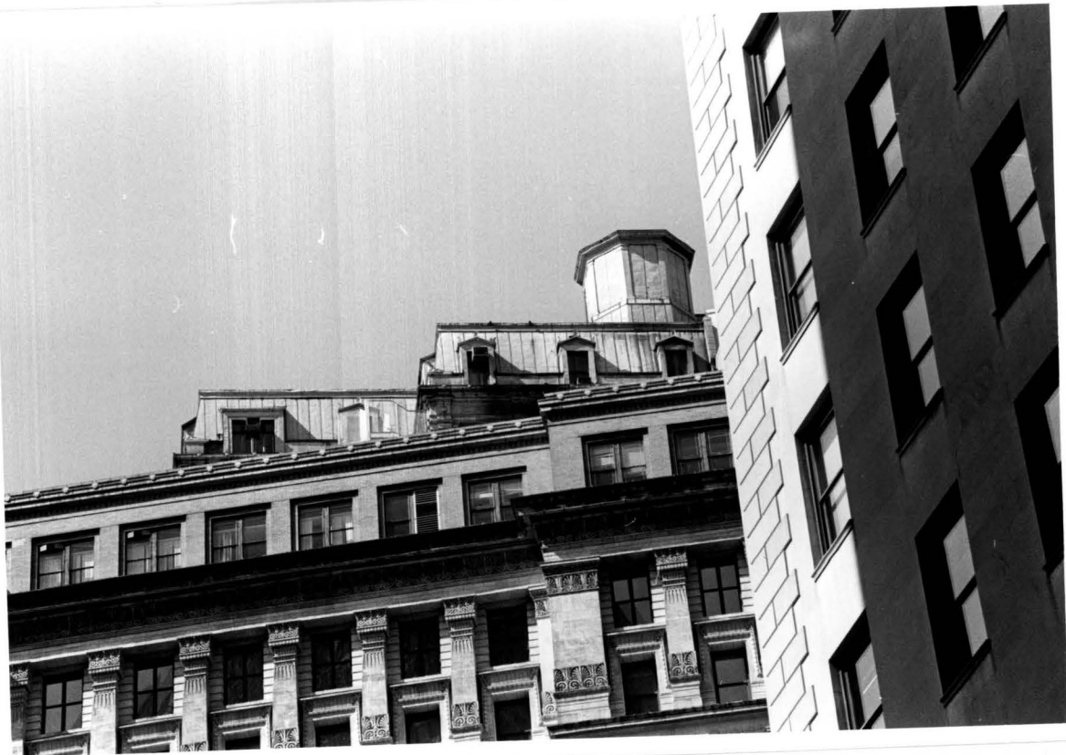
Fig. 10 Bowling Green Offices, Detail of rooftop additions facing Broadway
