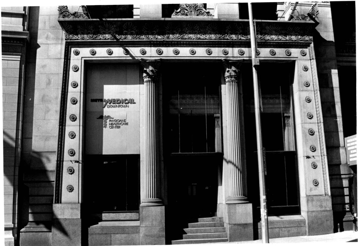
Fig. 8 Bowling Green Offices, South portico on Broadway
