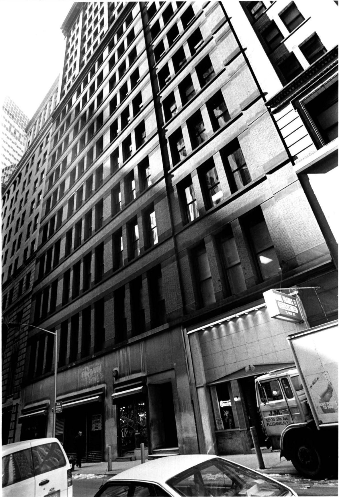
Fig. 13. Standard Oil Building, 26 Broadway, Manhattan. Northern portion of the New Street facade.
