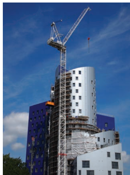
Picture 7.3 Student housing under construction in North End Road
