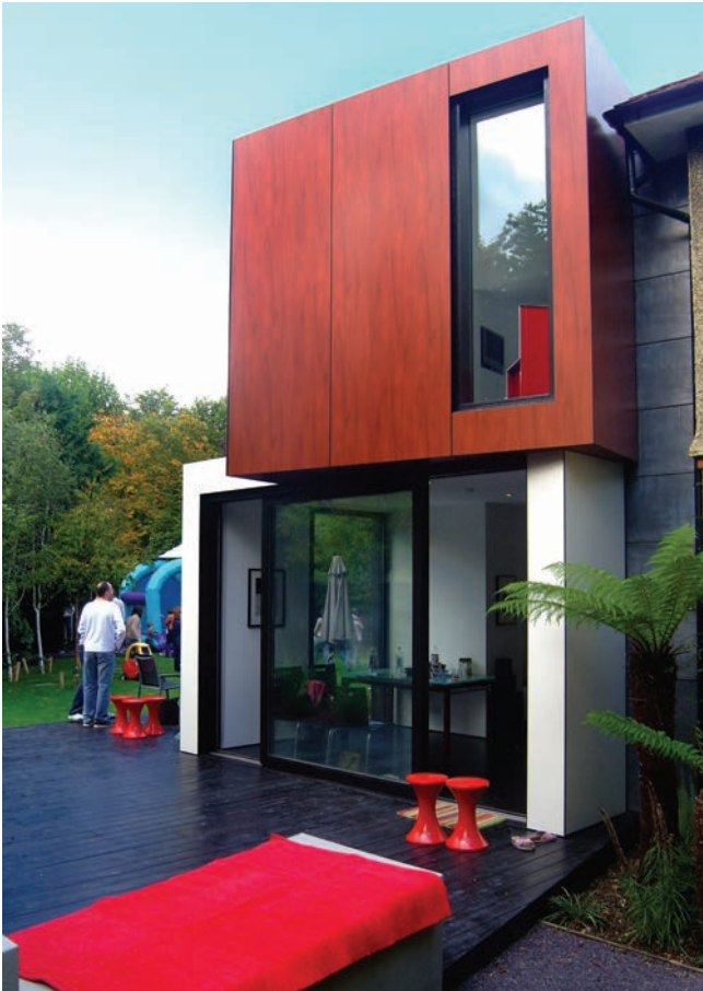
Picture 4.41 A well detailed contemporary home extension
