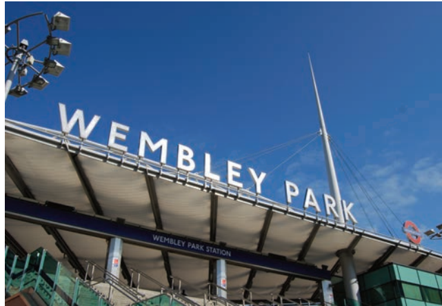
Picture 4.29 Wembley Park Station
