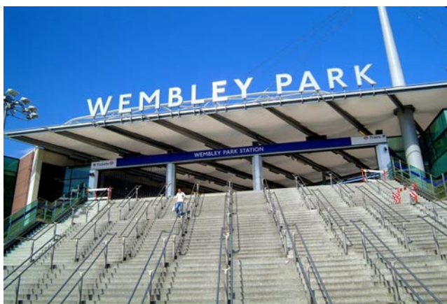
Picture 4.19 Wembley Park Station
