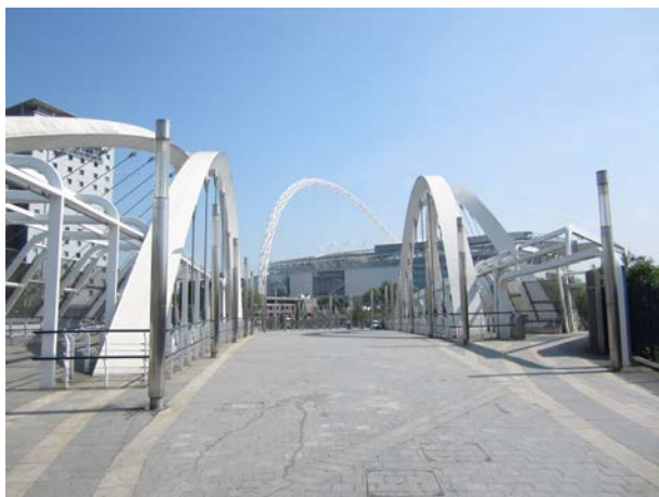
Picture 4.31 View of the Stadium from the White Horse Bridge
