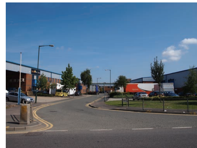
Picture 5.2 Towers Business Park, Carey Way
