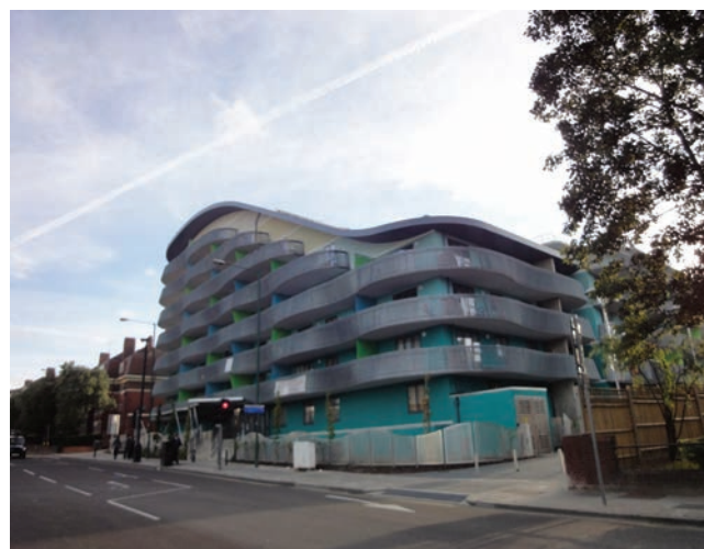
Picture 7.2 Ada Lewis House, Empire Way
