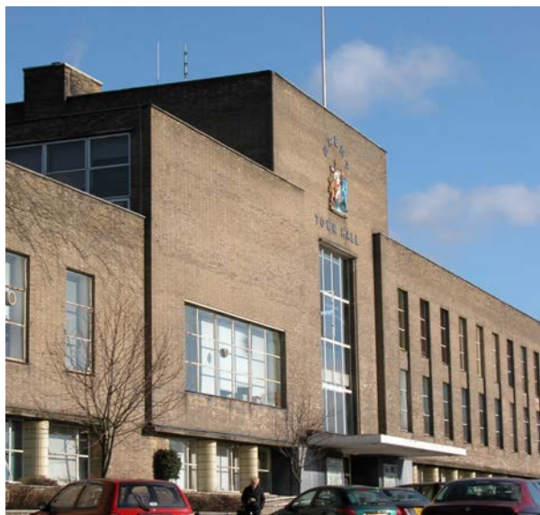
Picture 4.6 Brent Town Hall (Grade II)
