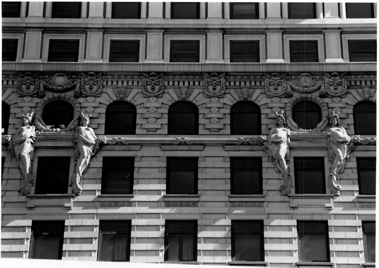
Top: Detail of the crowning cornice on Broadway Bottom: Detail of the sculptural ornament on the upper stories of the Broadway facade Photos: Carl Forster
