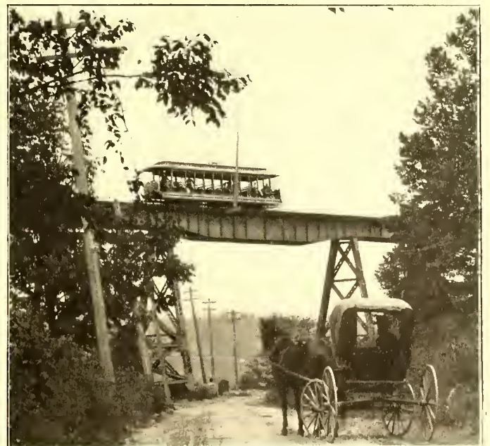
TYPICAL BRIDGE OVER HIGHWAY CROSSING
