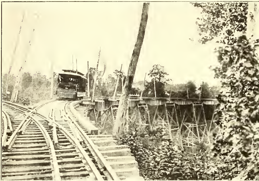
STEEL BRIDGE AT JUNCTION OF TWO DIVISIONS, SHOWING COMPLICATIONS OF THREE GAGES
