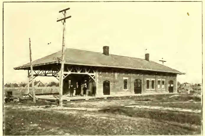
BETHEL SUB-STATION, PASSENGER AND FREIGHT HOUSE
