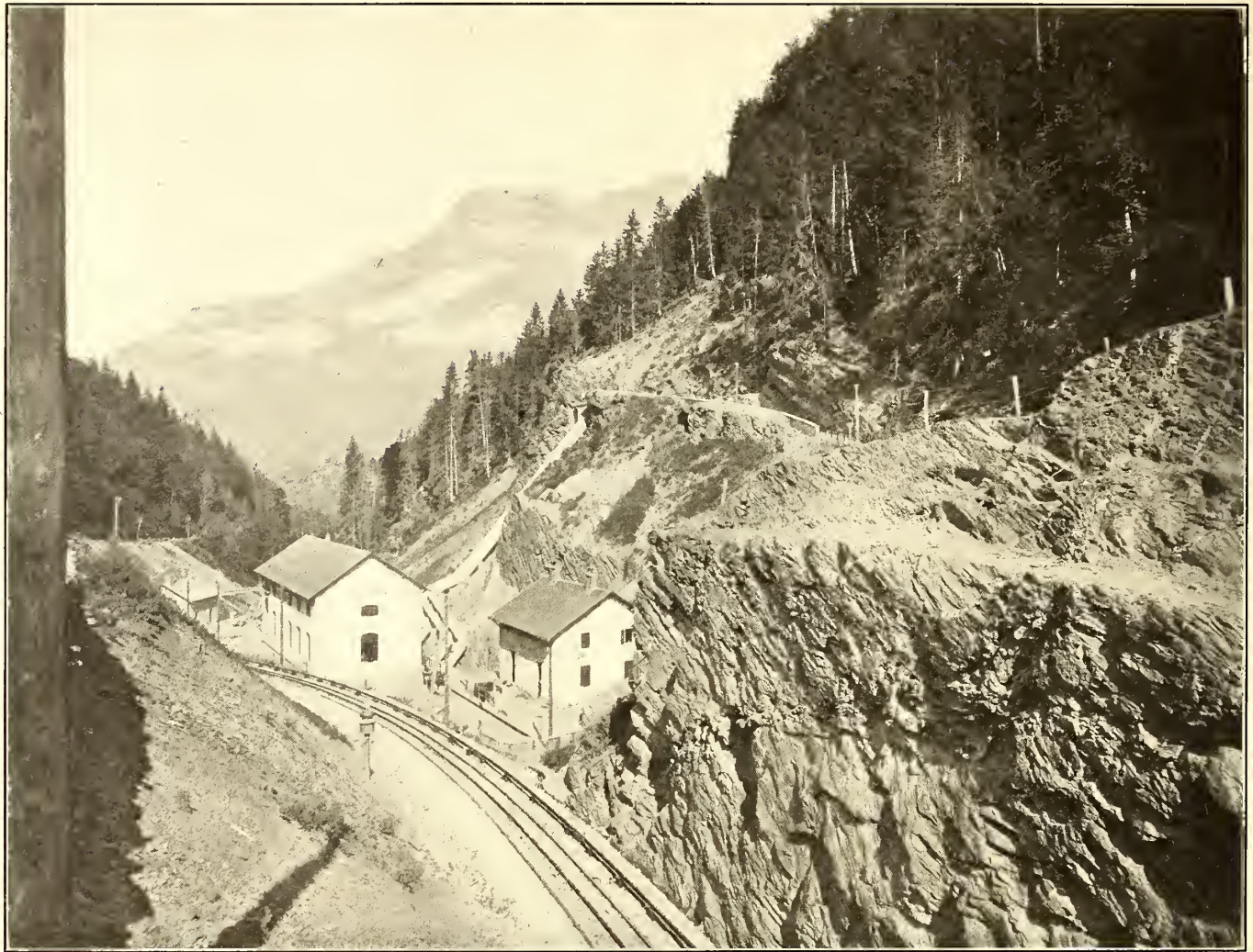
HYDRAULIC POWER STATION AT SERVOZ
