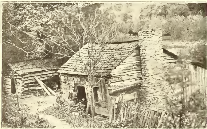
PRIMITIVE HOME DIRECTLY UNDER LONG TRESTLE OF CINCINNATI, GEORGETOWN & PORTSMOUTH RAILWAY
