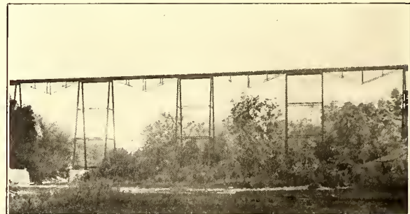
STEEL TRESTLE 110 FT. ABOVE WATER
