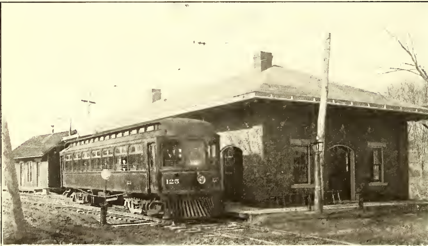
MOUNT WASHINGTON SUB-STATION AND PASSENGER DEPOT
