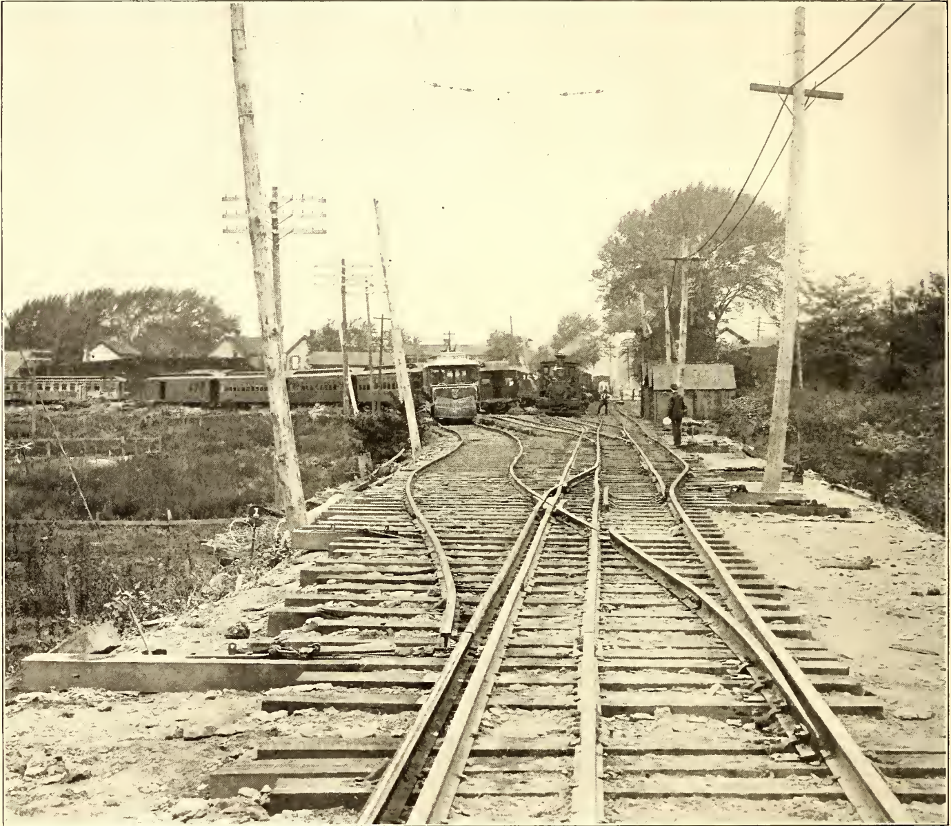
YARDS OF CINCINNATI, GEORGETOWN & PORTSMOUTH RAILWAY, SHOWING COMPLICATIONS OF TRACKS CAUSED BY THREE GAGES
