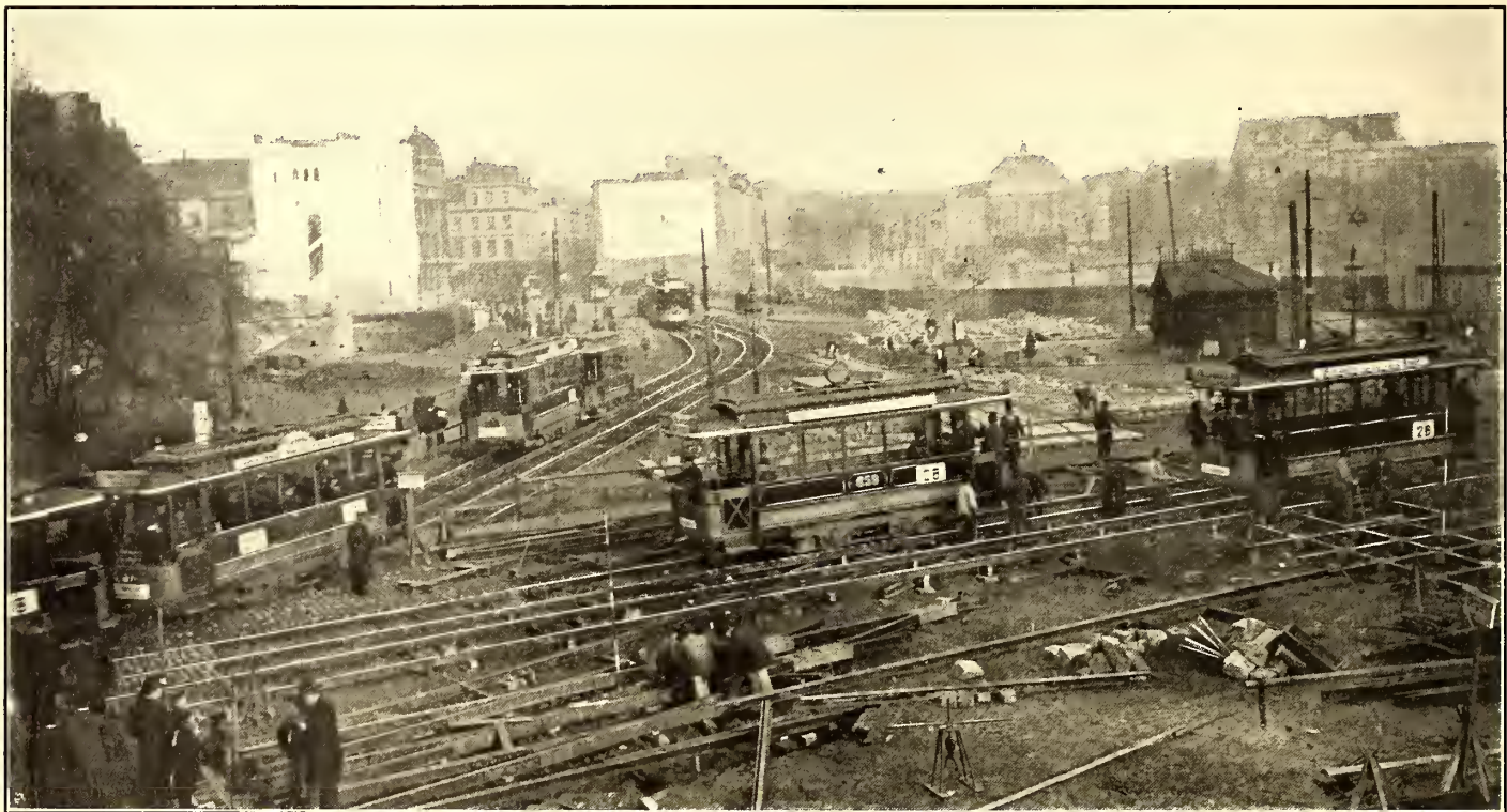
INTERESTING TRACK WORK IN HAMBURG
