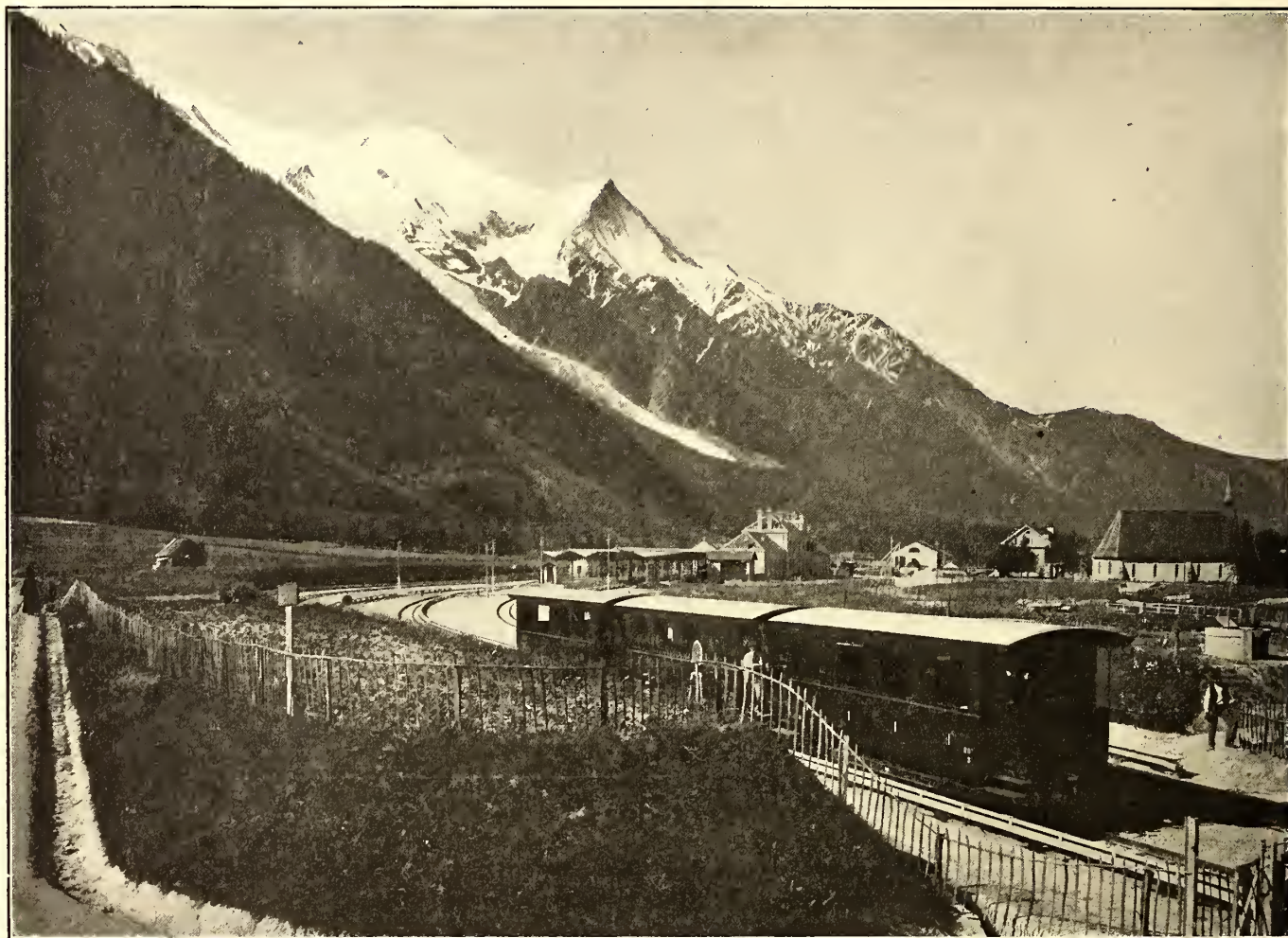
GENERAL VIEW OF ELECTRIC TRAIN, STATION AT CHAMONIX AND MOUNT BLANC
