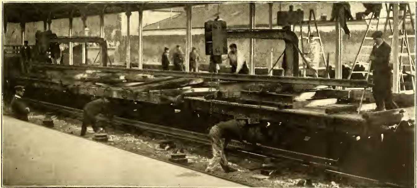
METHOD OF LAYING THIRD RAIL
