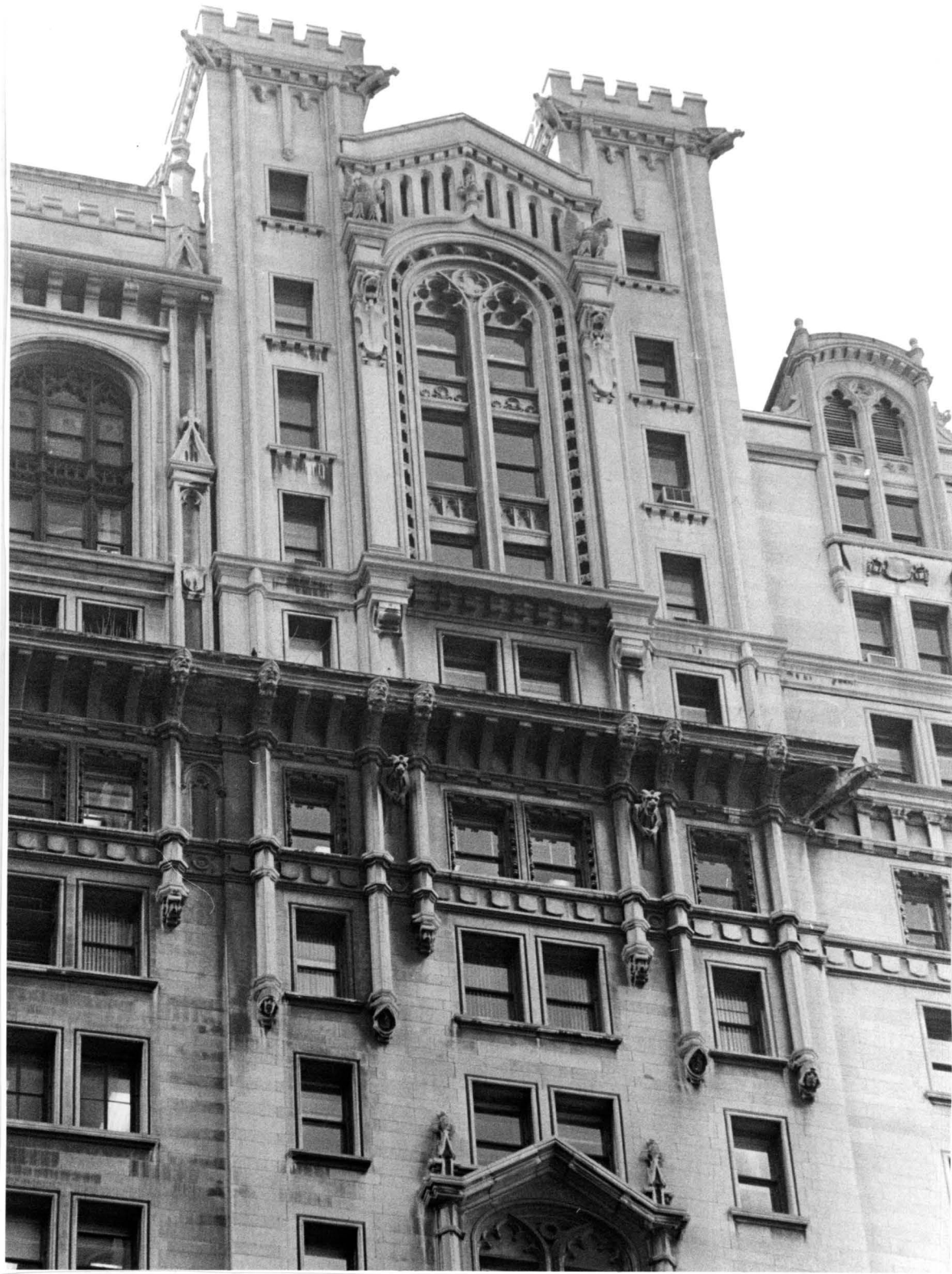
U.S. Realty Building Detail, northern elevation, showing window bay and parapet
