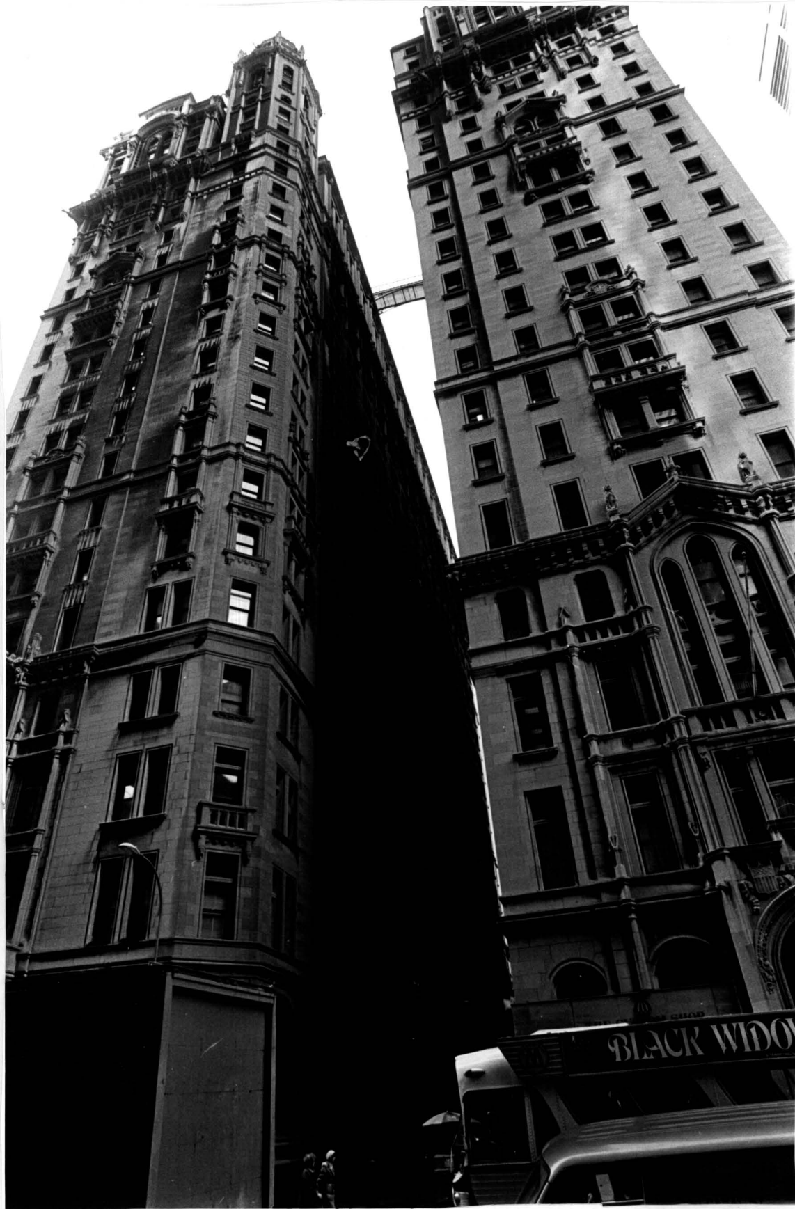
U.S. Realty Building Broadway facade, with the Trinity Building on the left
