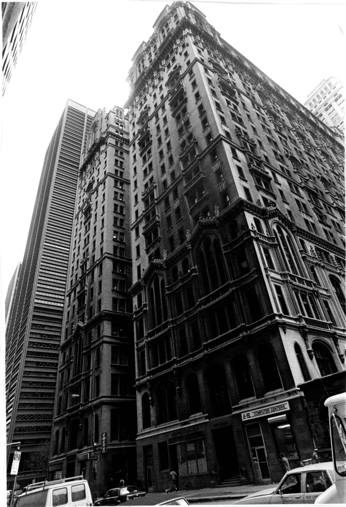
U.S. Realty Building Trinity Place elevation, with the Trinity Building on the right
