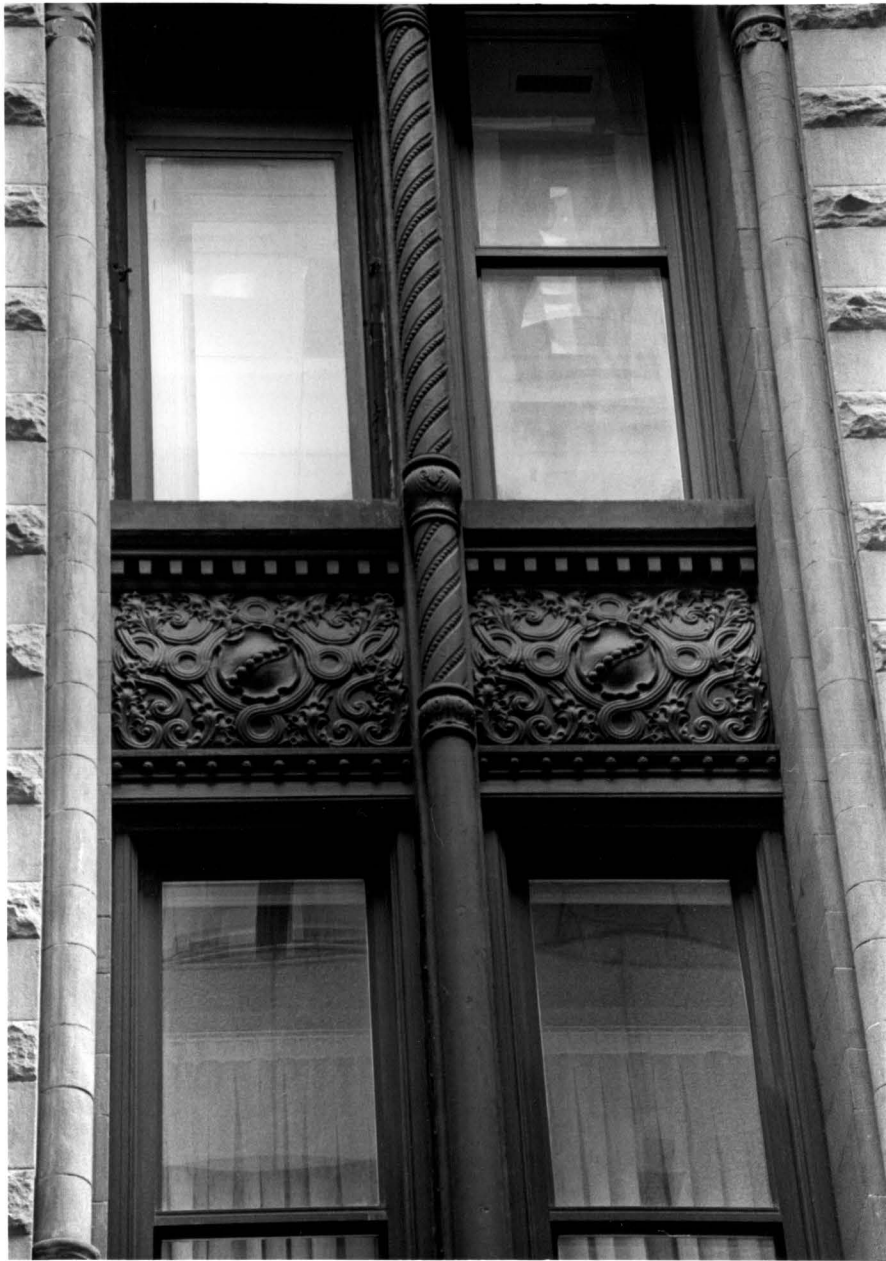
56-58 Pine Street Building, spandrel detail, 2nd-3rd stories, Pine Street facade
