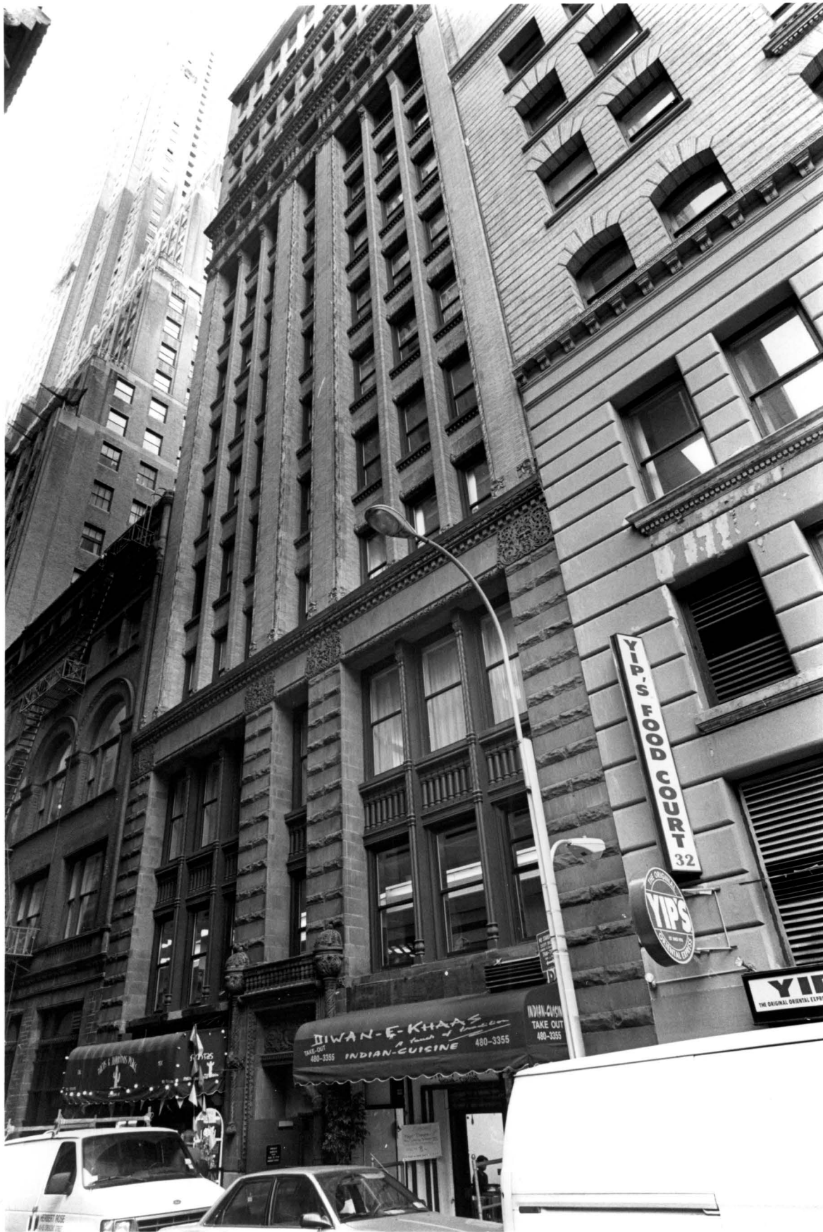
56-58 Pine Street Building, Cedar Street facade
