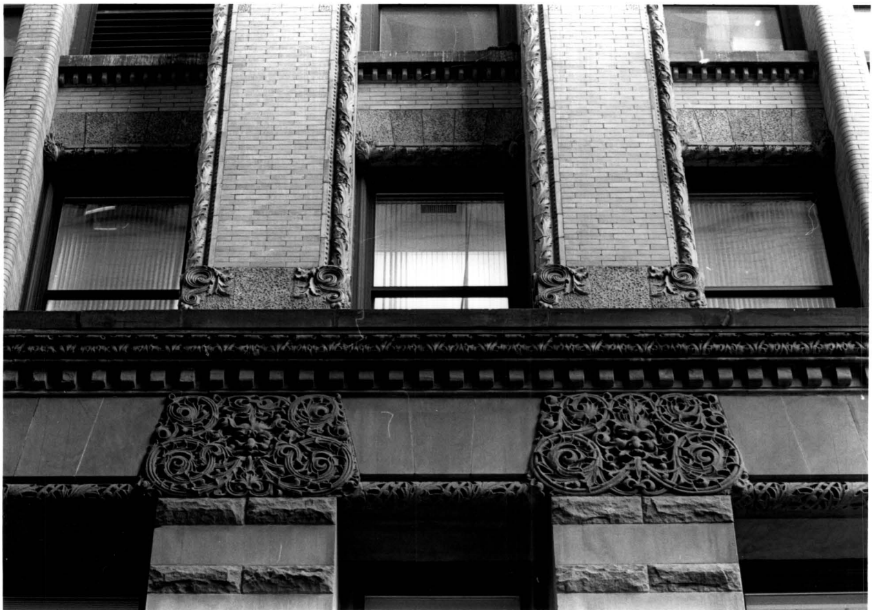
56-58 Pine Street Building, terra-cotta detail, 3rd-4th stories, Cedar Street facade
