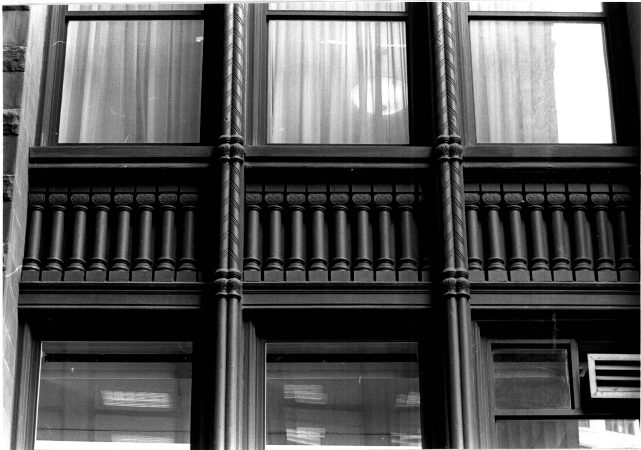
56-58 Pine Street Building, spandrel detail 2nd-3rd stories, Cedar Street facade
