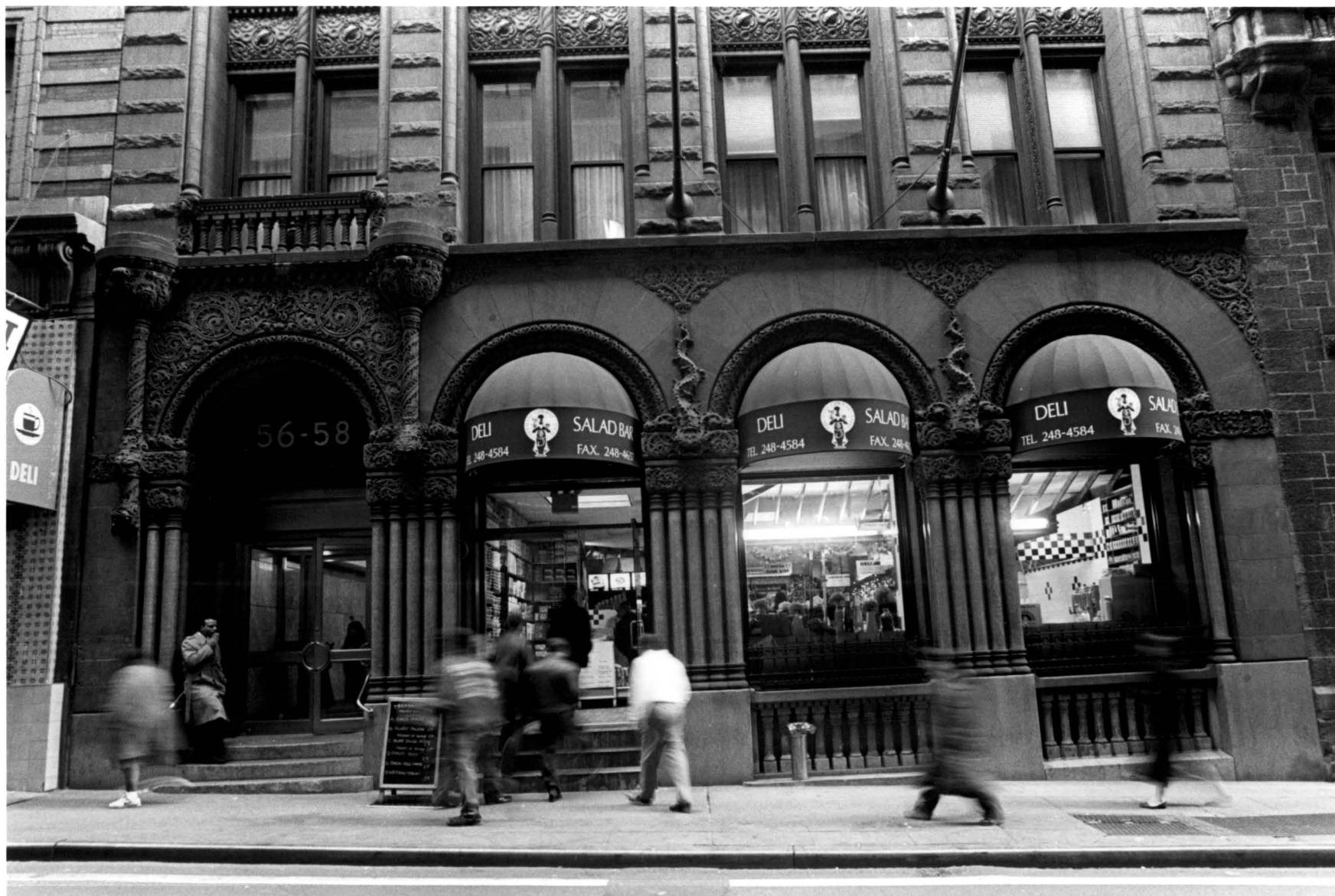
56-58 Pine Street Building, ground story, Pine Street facade
