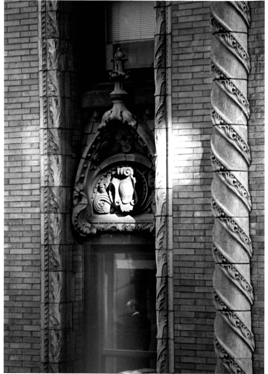
56-58 Pine Street Building, hood detail, 9th story, Pine Street facade
