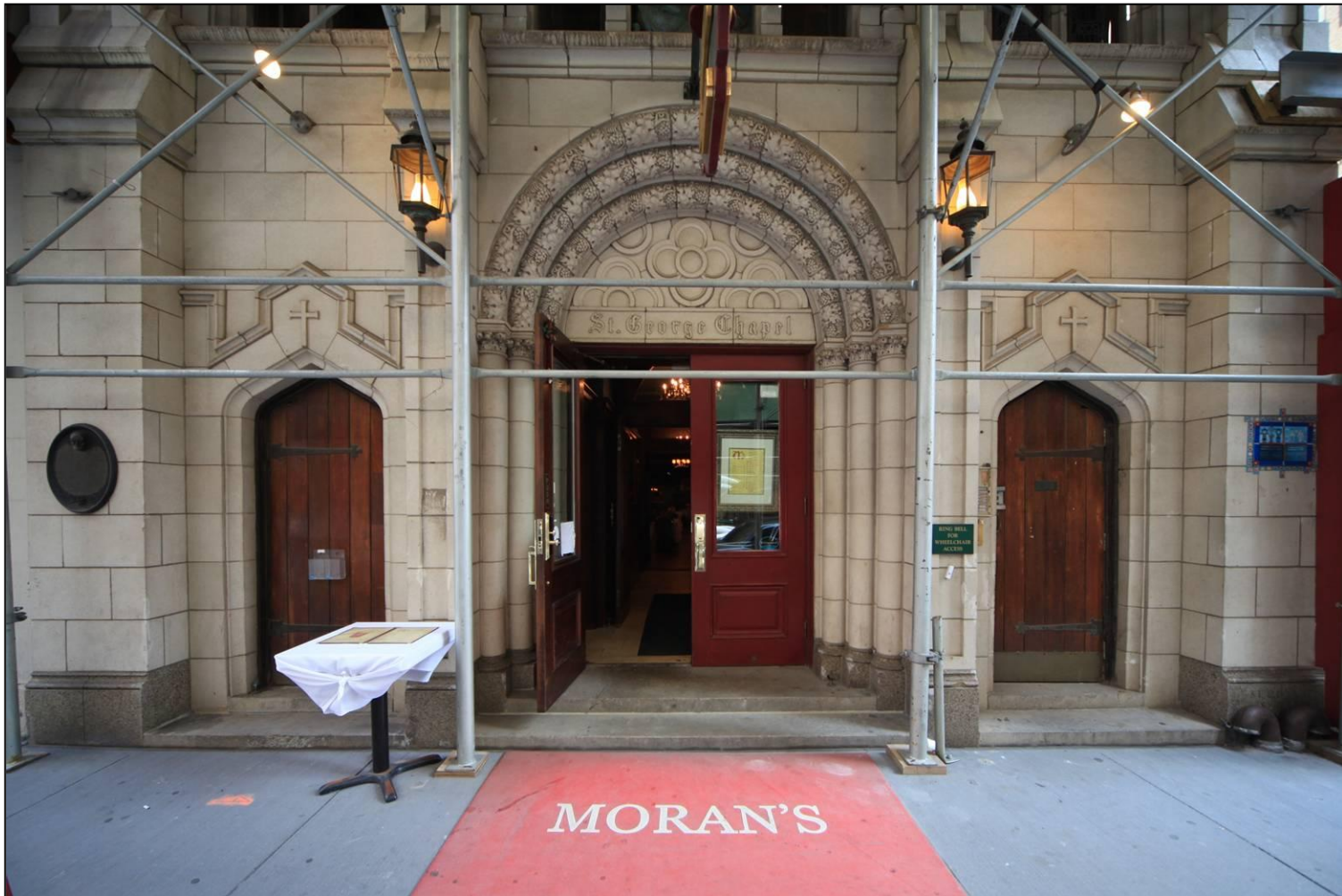
(Former) St. George's Syrian Catholic Church, 103 Washington Street, Manhattan First floor, main facade Photo: Christopher D. Brazeo, 2009
