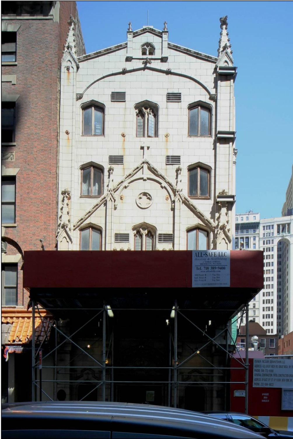
(Former) St. George's Syrian Catholic Church 103 Washington Street, Manhattan Main facade Photo: Christopher D. Brazee, 2009
