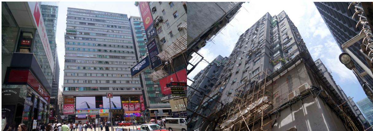
Fig. 11 Chungking mansions in Nathan road as a highly dense mixed use building complex.
