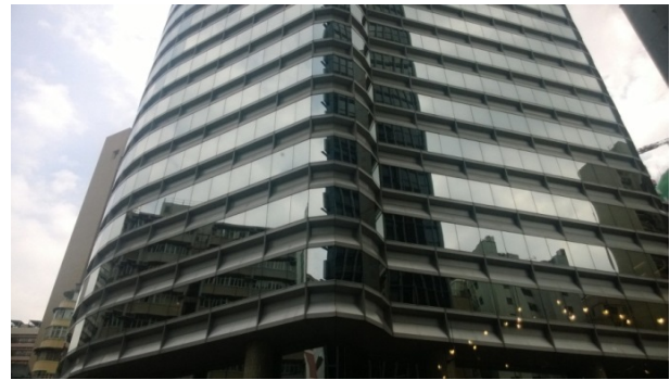
Fig. 20 Continuous bay windows in an office building (Tai Yau Plaza) completed in the 80s.
