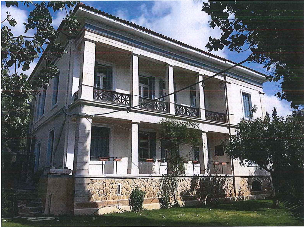
The 'Upper House', original home of the BSA in 1886; exterior restored through a generous donation in Summer 2017
