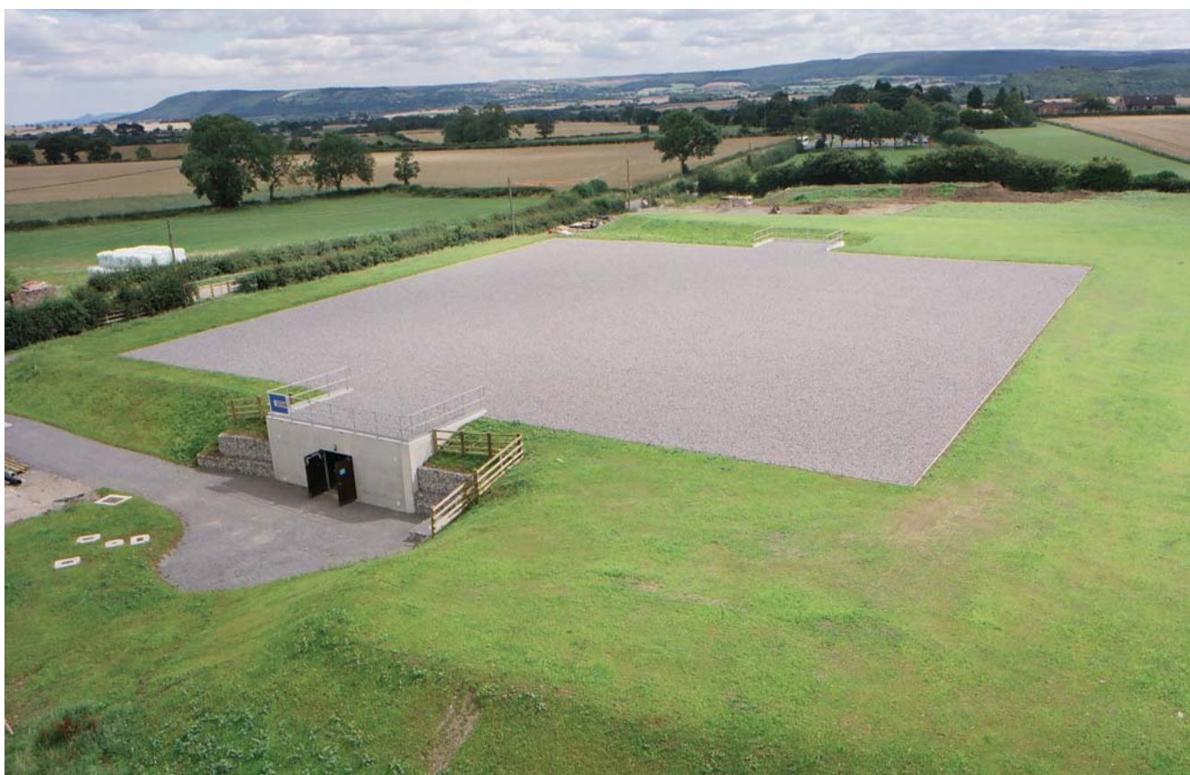
Aerial view of completed increased capacity at Bullamoor Service Reservoir
