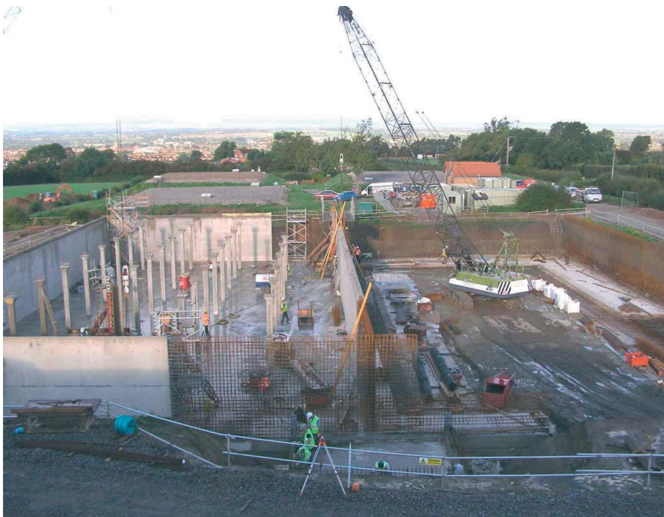
Tank 4 under construction
