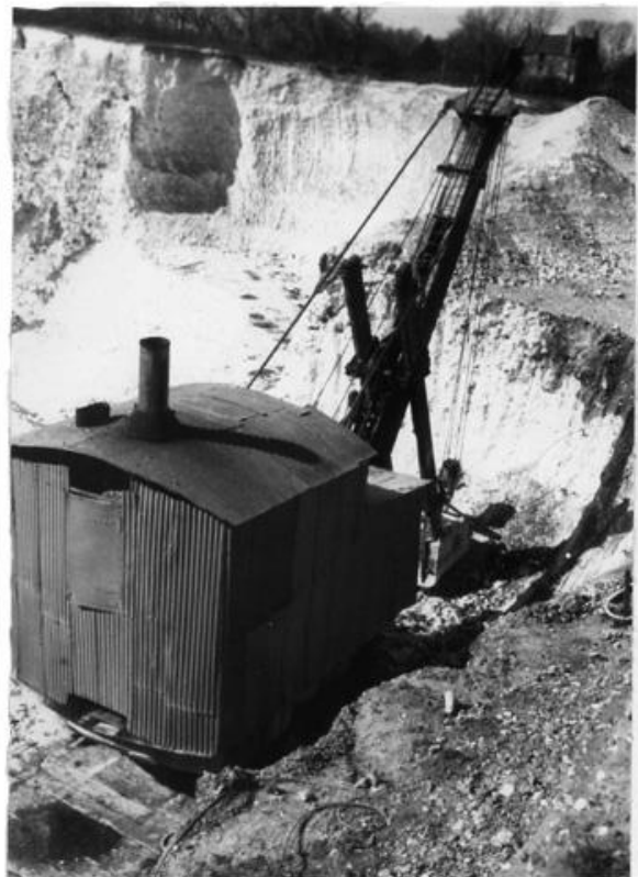
Excavating chalk from the quarry near All Saints Church
