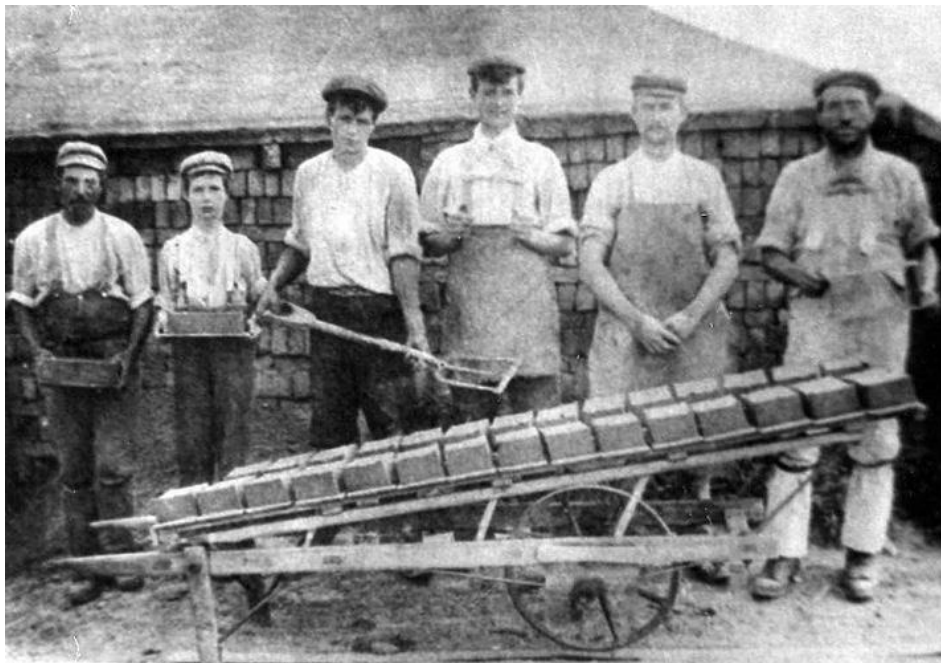
A brickmaking gang at Rainham in 1890 standing in front of a hack. Note the moulds, large cuckle and brick barrow.
