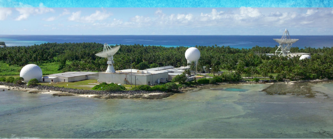
The Kiernan Re-entry Measurement Site radars on Roi-Namur.
